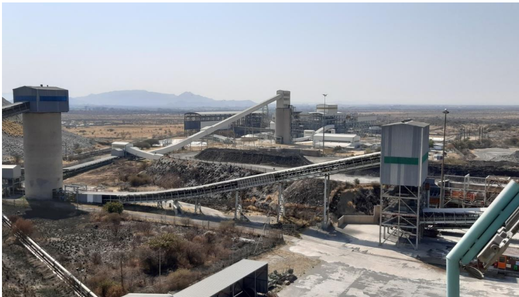
Figure 6: Platinum plant ore transfer conveyors
