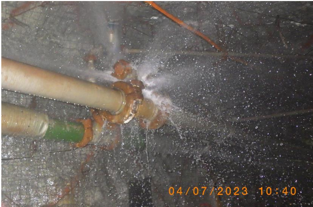
Figure 46: Identified water-use inefficiency.
