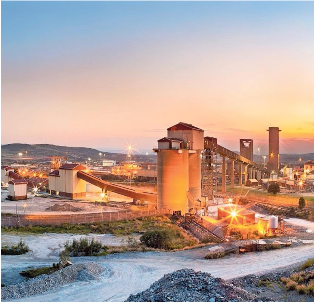
Figure 1: Typical mining shaft in South Africa 1 .
