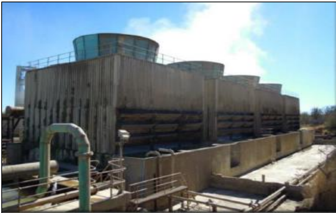
Figure 19: Example of pre-cooling towers [29].
