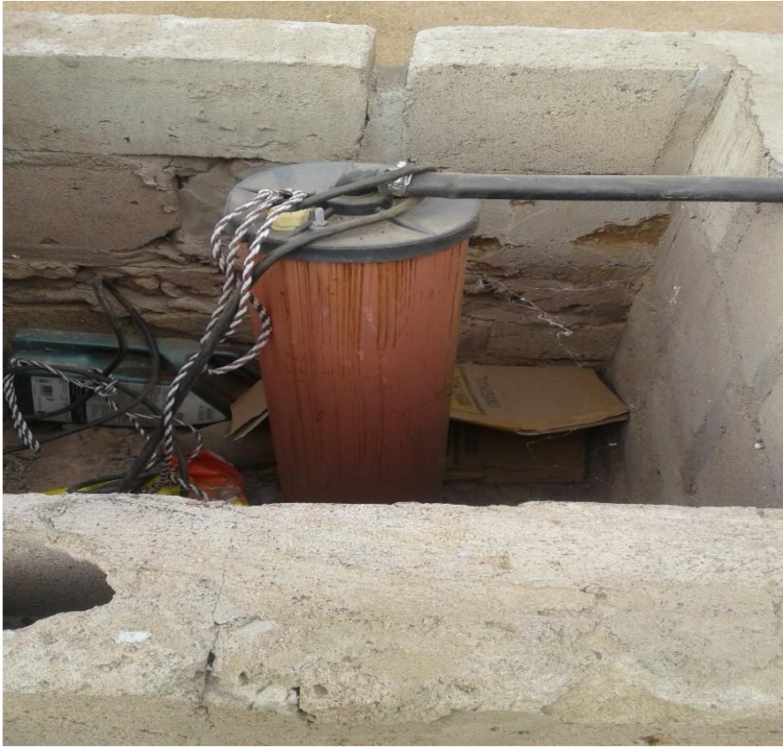
Photo 6: Enclosed borehole where water level cannot be measured
