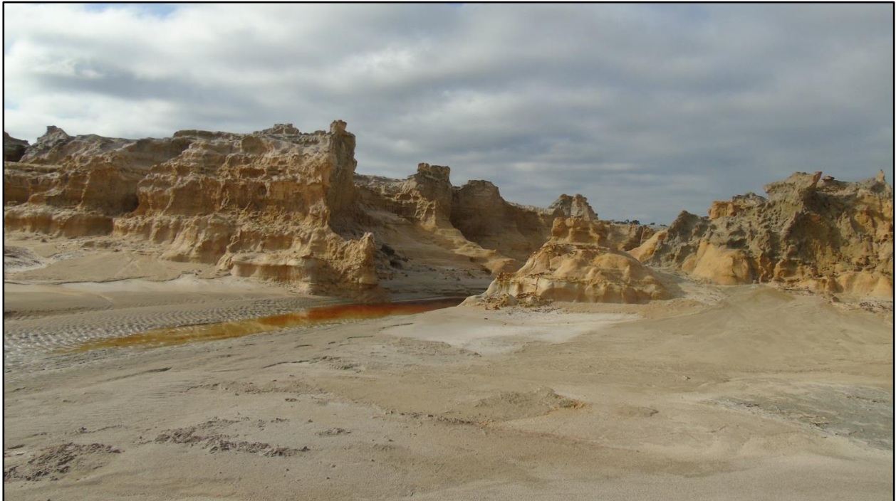
Figure 5: A photograph of AMD seepage at a gold TSF in South Africa. Photograph taken by Daniell (2016), with permission.
