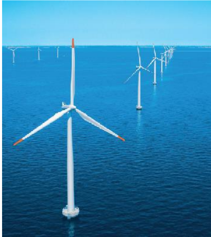
Figure 6.2: Horizontal Axis Wind Turbine (HAWT)
