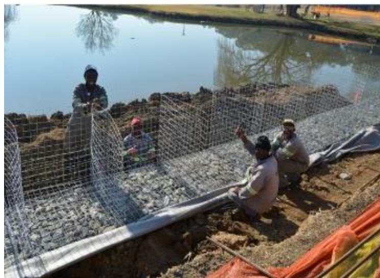
Photo 5.6: The construction of gabions at Dam 4 to limit erosion (VAAL eNUUS, 2017)
