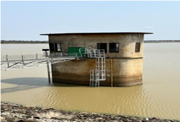
Figure 8: Nsami dam at an average dam level.
