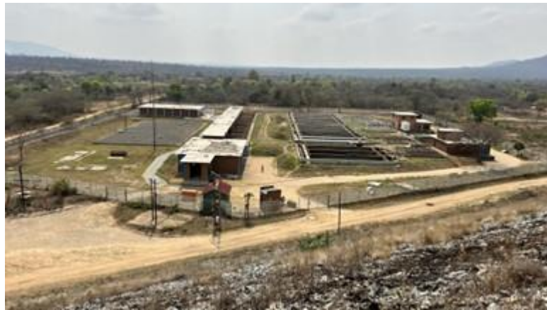
Figure 9: Middle Letaba WTW operating below capacity due to insufficient water.
