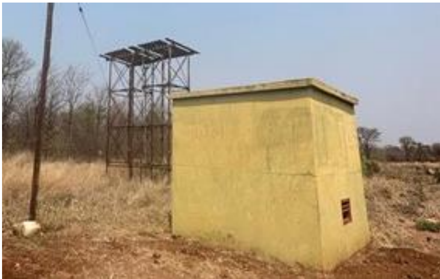
Figure 16: Transformer meant to energise the borehole was missing.
