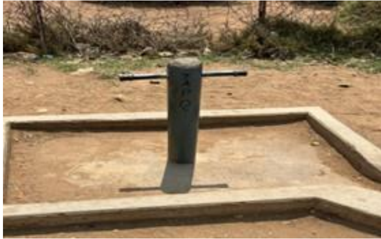
Figure 15: Vandalised water tap by community members.
