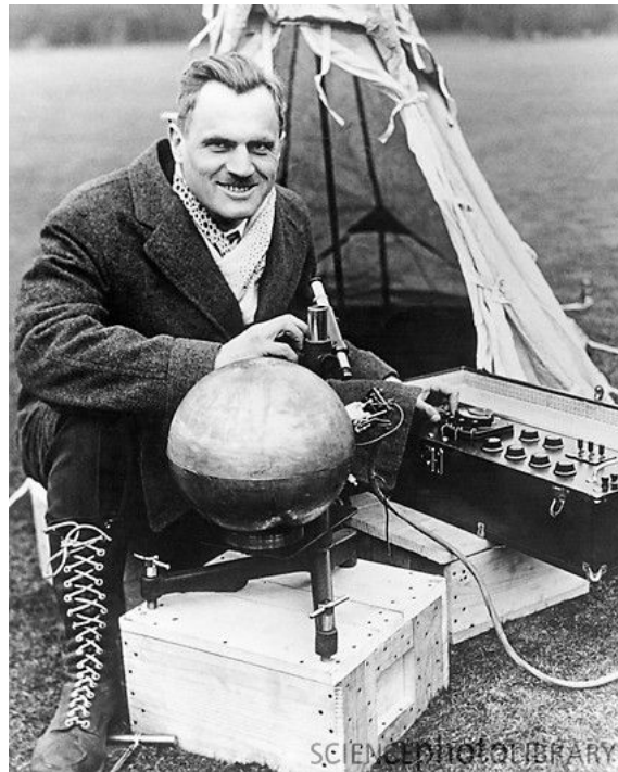
Figure 1.2.: Arthur Holly Compton with a model C cosmic ray ionization chamber (American Institute of Physics/Science photo library).
