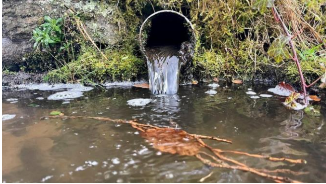
Untreated wastewater in dams
