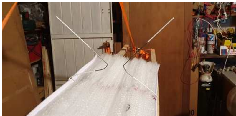
Figure 4-6: Arc horns on top of capacitor stack.
