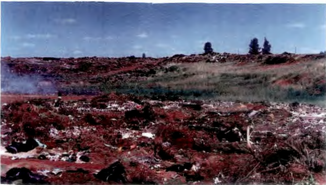
FIGURE 20 STILFONTEIN LANDFILL SITE – 2001 – Waste deposition – NO trenches or cells used for deposition, waste not covered on daily basis, fires not controlled
