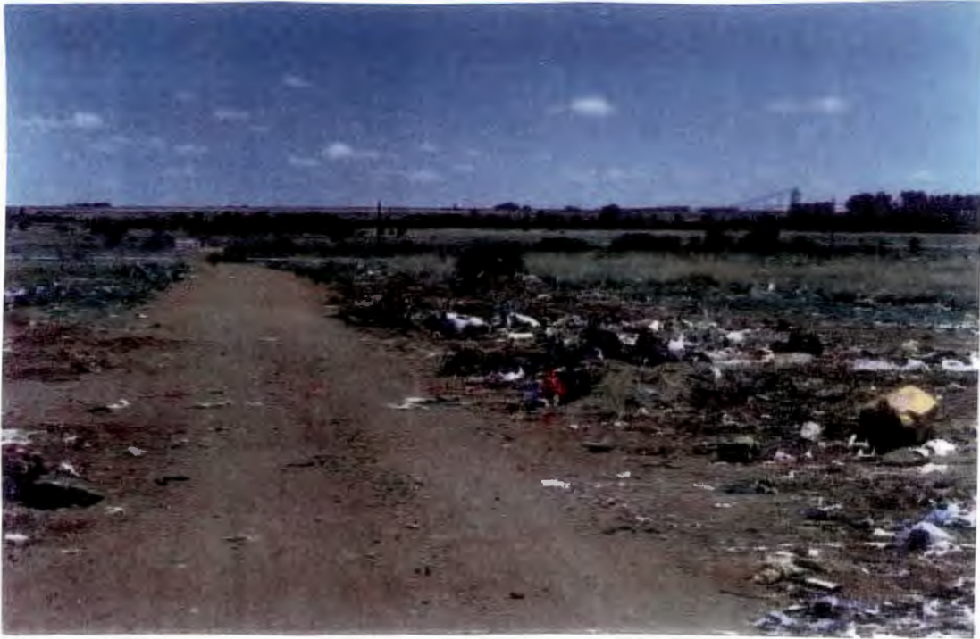
FIGURE 12 ORKNEY LANDFILL SITE – 2000 – Condition of the road and traffic control – access roads road to site maintained, two traffic possible, unsurfaced road regularly graded
