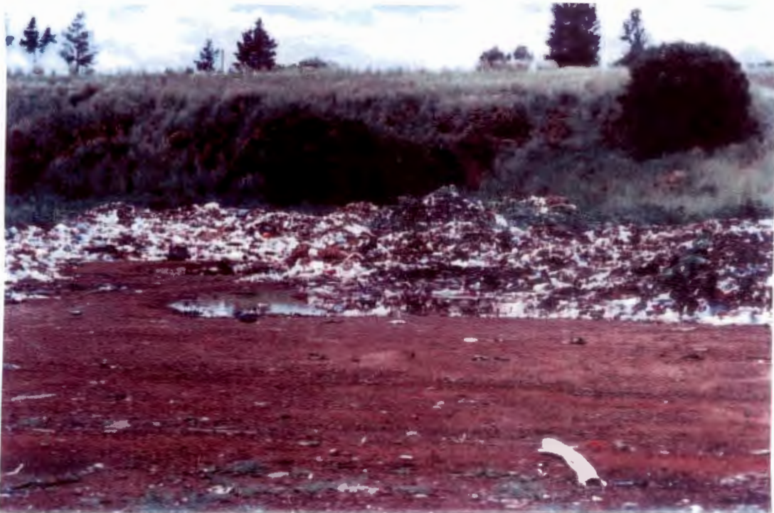
FIGURE 23 STILFONTEIN LANDFILL SITE – 2001 – Drainage – runoff water not diverted from the site
