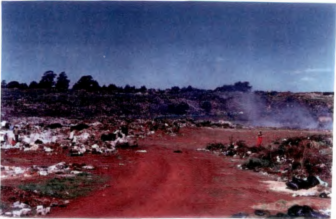
FIGURE 14 THE STILFONTEIN LANDFILL SITE – 2000 – Condition of the road and traffic control – Access road to the site maintained, waste can reach the working face with minimum inconvenience. Two way traffic possible in all weather conditions, regularly graded
