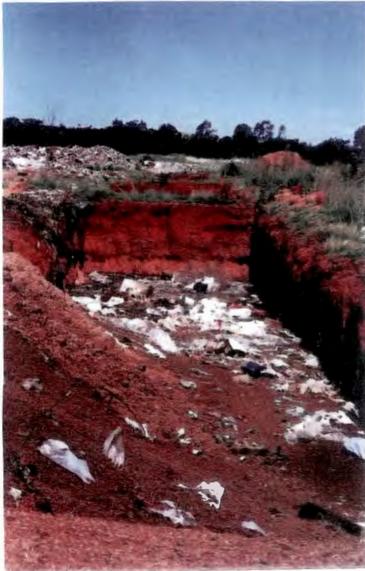
FIGURE 18 KLERKSDORP LANDFILL SITE – 2000 – Waste deposition – trenches on site
