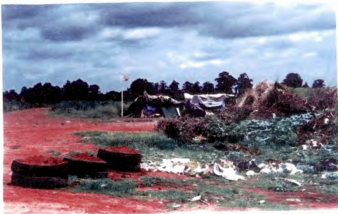
FIGURE 11 STILFONTEIN LANDFILL SITE – 2001 – Site access – site boundaries demarcated by tyres
