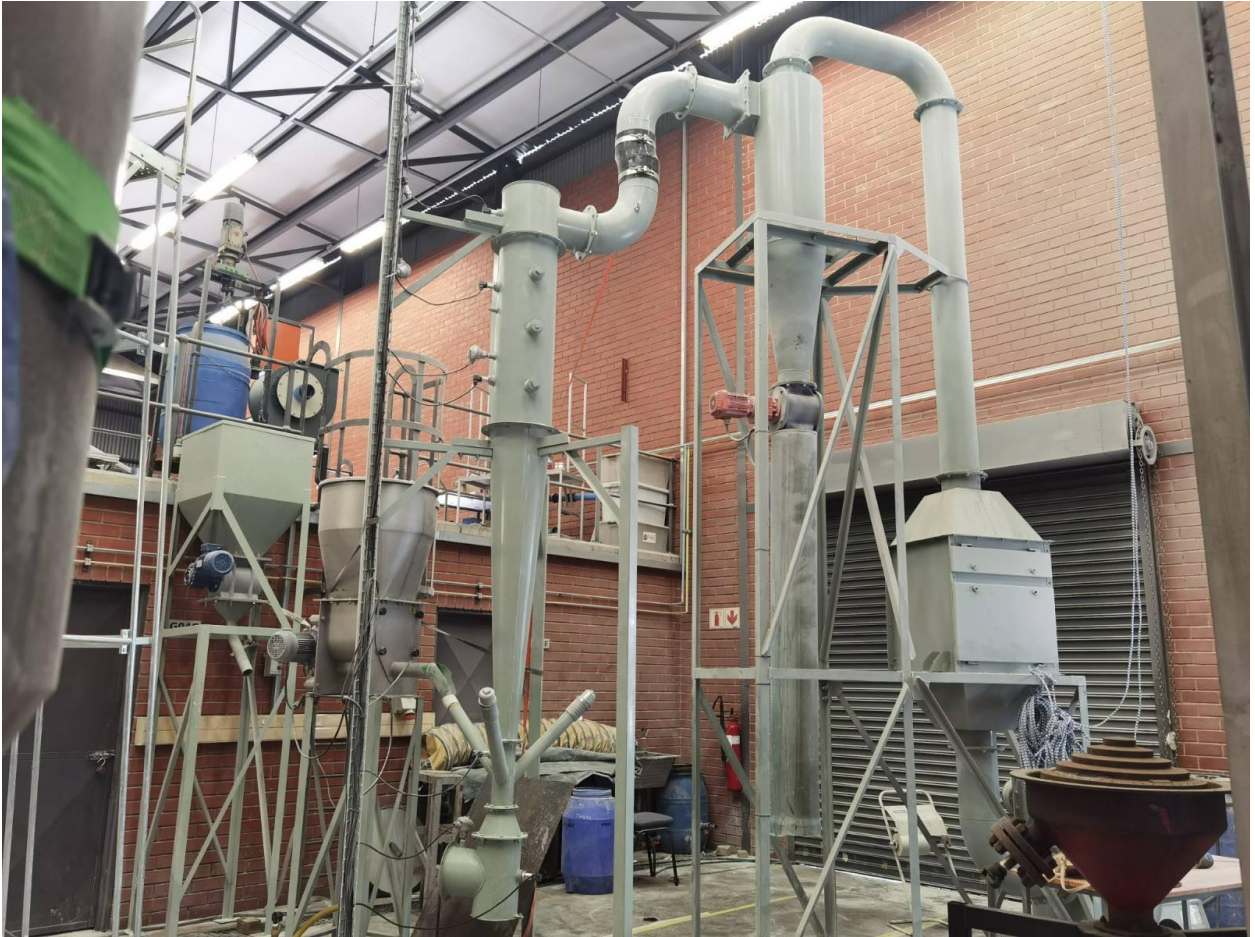
Figure M2: Riser when only one cylindrical section was installed
