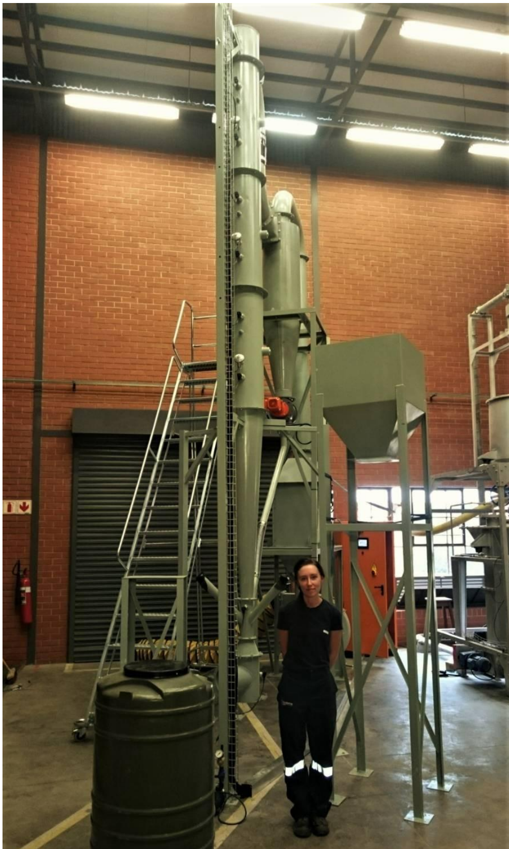
Figure M1: Riser during its construction
