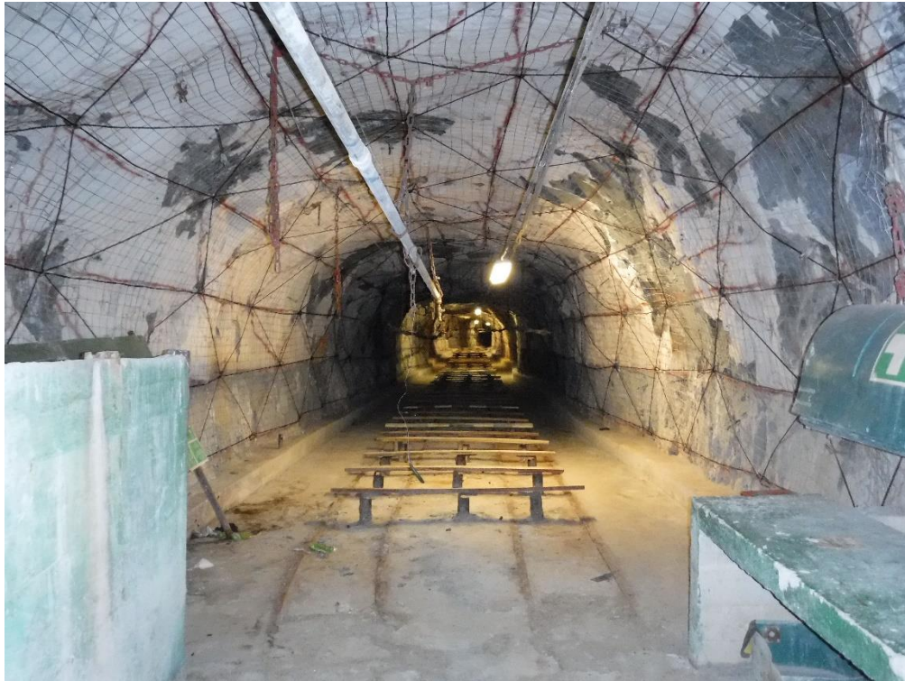
Figure 9: Underground refuge bay 3
