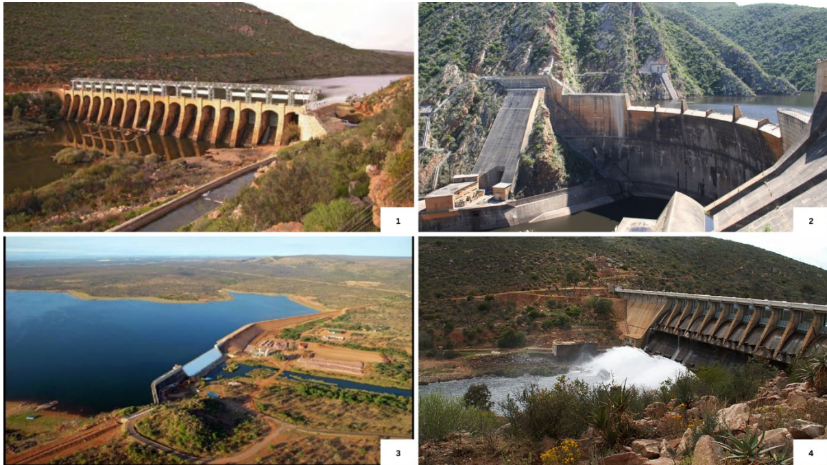
Figure 2-1: Four most prominent types of dams in South Africa: 1- Buttress dam; 2- Arch dam; 3- Embankment dam; 4- Gravity dam 58
