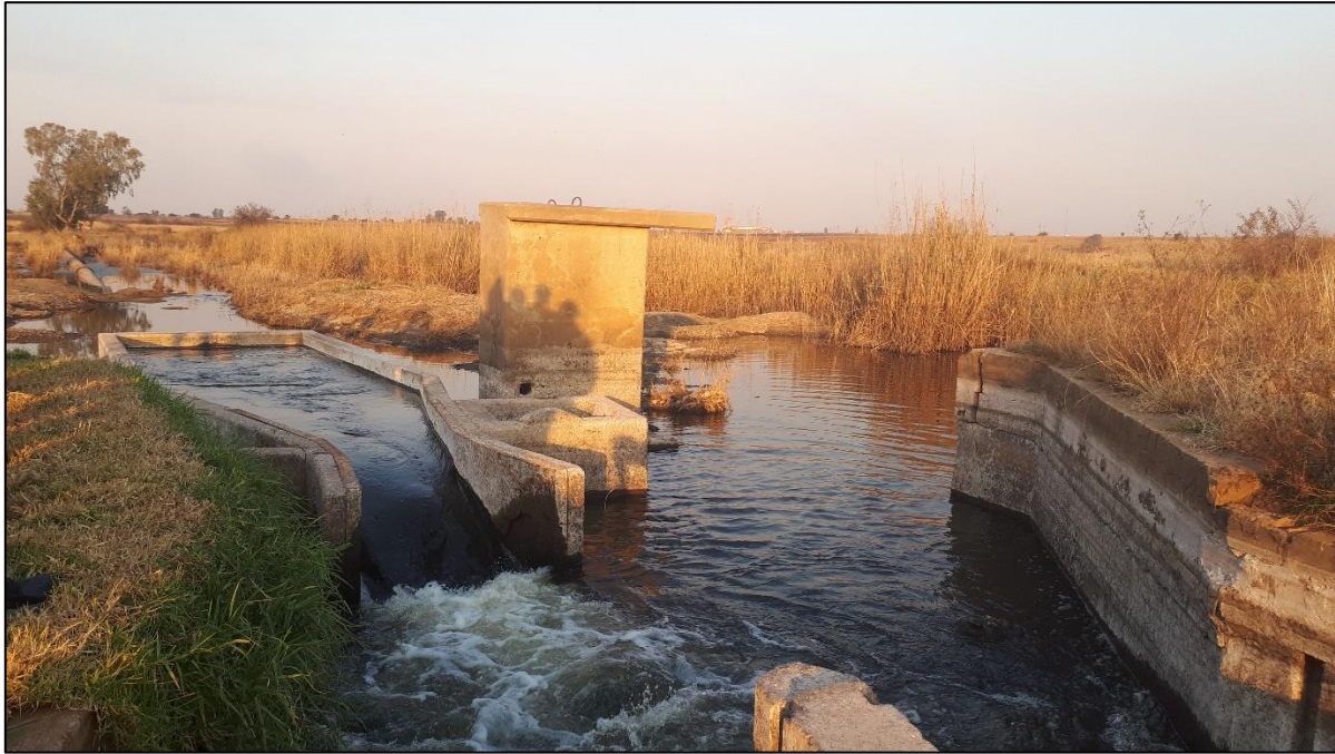
Figure 19: Open channel inlet for the Wonderfonteinspruit 1m diversion pipeline (Kriel, 2019).
