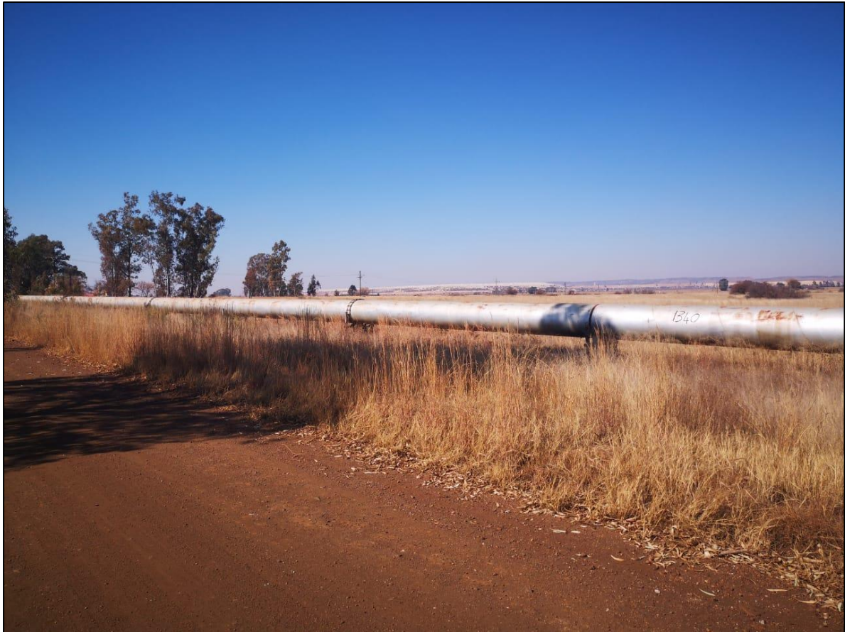
Figure 20: 1m diameter conveying pipeline (Kriel, 2019).
