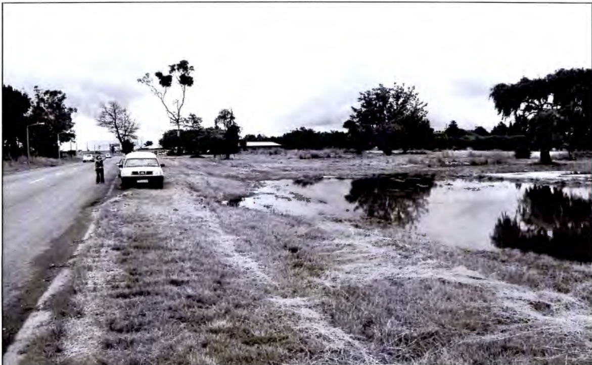
Figure 4: Small surface dam of raw sewage near the D field potable water abstraction boreholes and 300m from the municipal offices in Delmas
