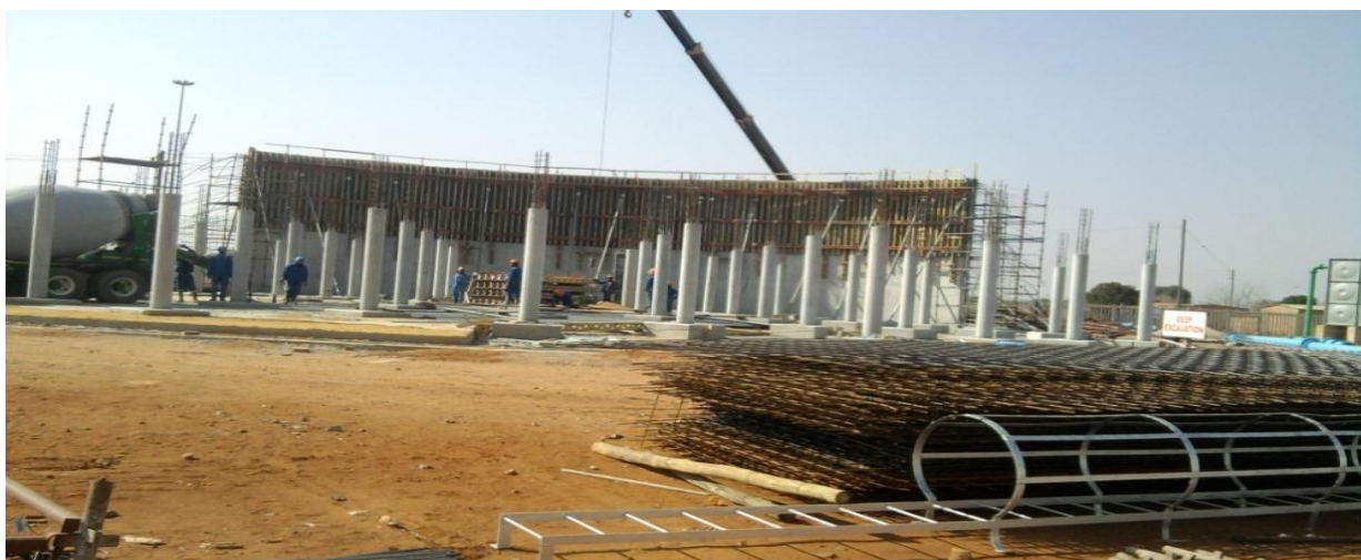
Figure 12: Construction of the new water reservoir in Khuma extension 8 (Researcher's personal library)
