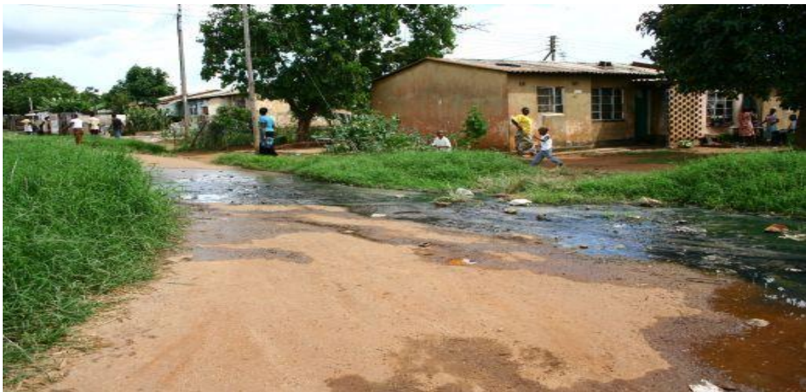
Figure 3: Sewage-overflow in some parts of Khuma Township (Researcher's Personal Library)
