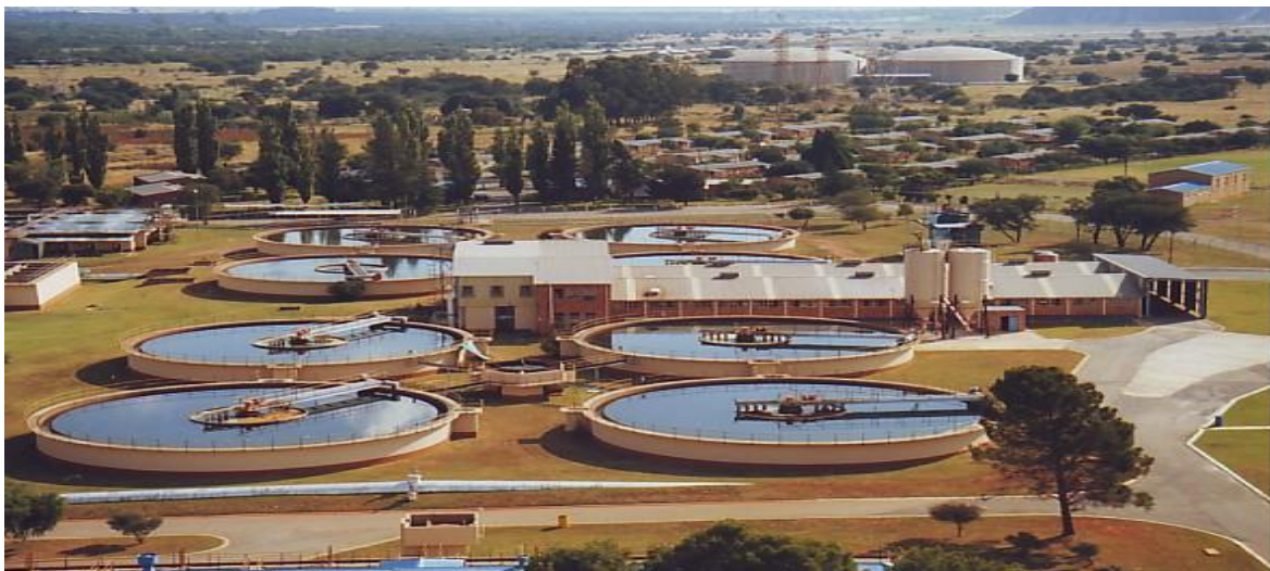
Figure 1: Photograph of Midvaal Water Company Treatment Site (Midvaal Water Company, 2010).
