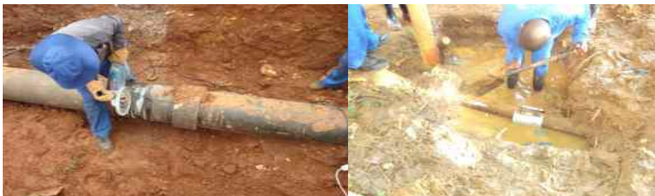
Figure 10: Maintenance of water pipes in the Klerksdorp area. (Researcher's Personal Library)
