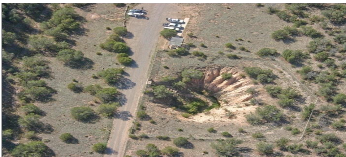
Figure 6: Sinkhole due to underground cavities. (DWA, 2009)
