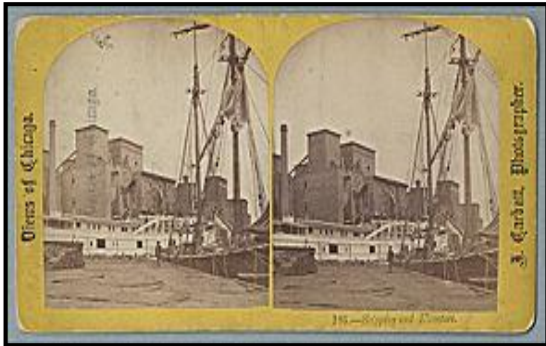
Figure 2.4 Elevators, bunkers and ships on the Chicago river (Gregory, 2005)
