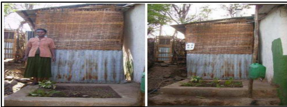
Figure 2.3: The Fossa Alterna, plants planted on the filled pit
