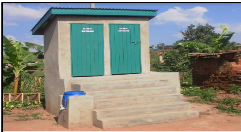
Figure 2.2: Ventilated Improved Double Pit latrine, Kampala, Uganda
