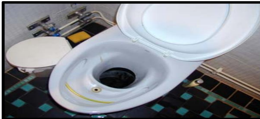
Figure 2.1: Dry urine-diversion toilet
