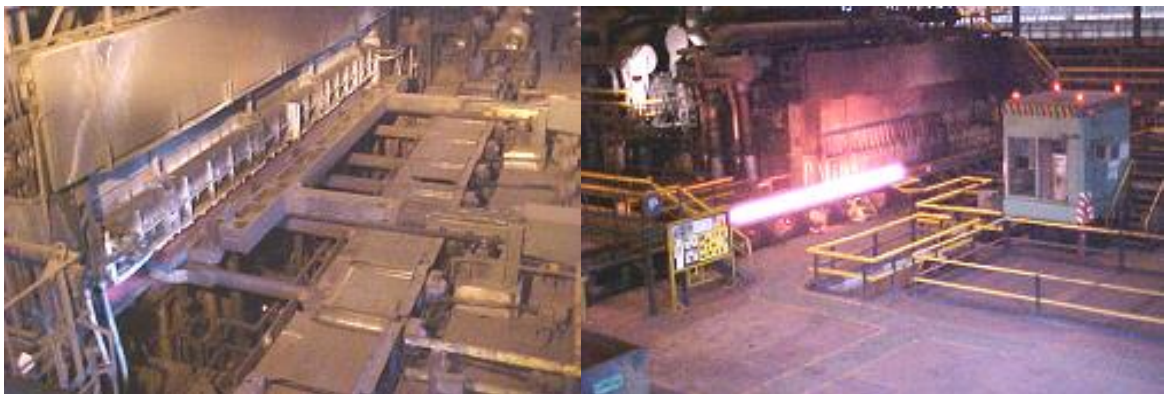
Figure 4-3: Mill 2 reheating furnace
