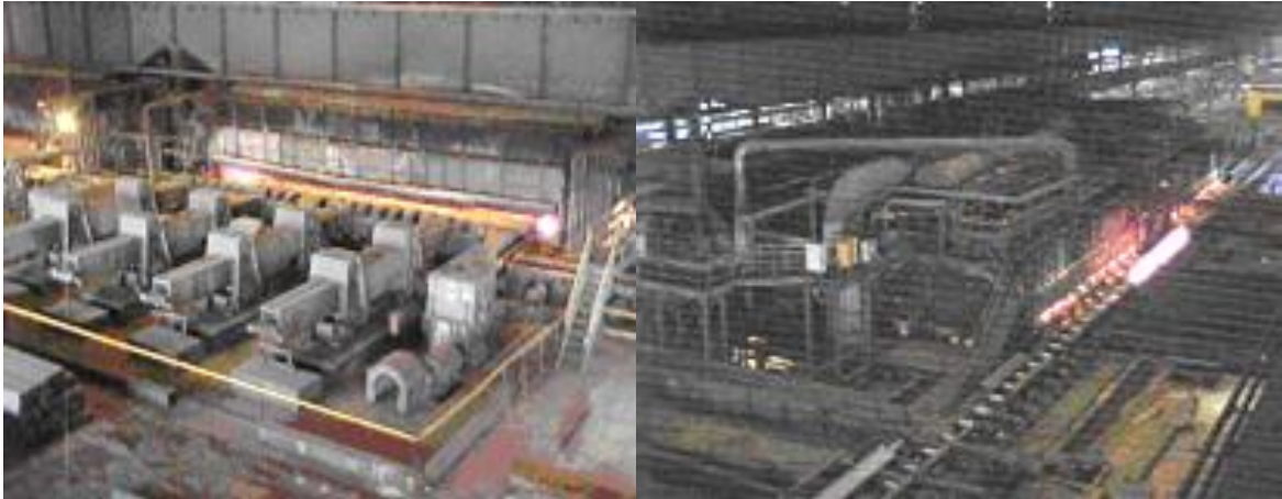
Figure 4-2: Mill 1 reheating furnaces
