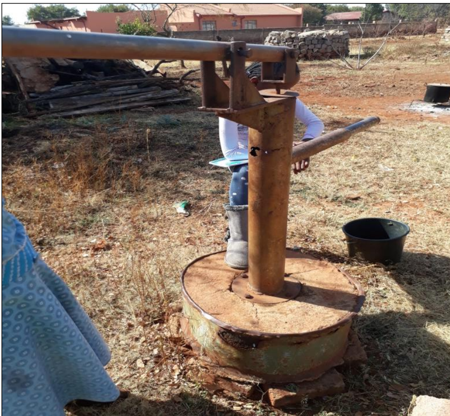
Figure 3-1: Borehole no longer in use
