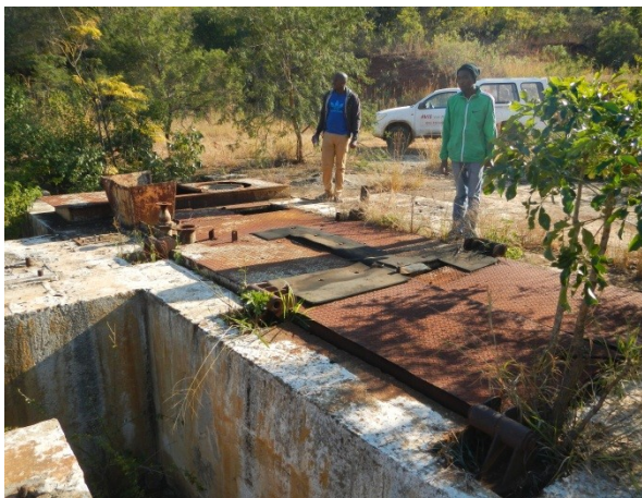
a) Vertical shaft.
