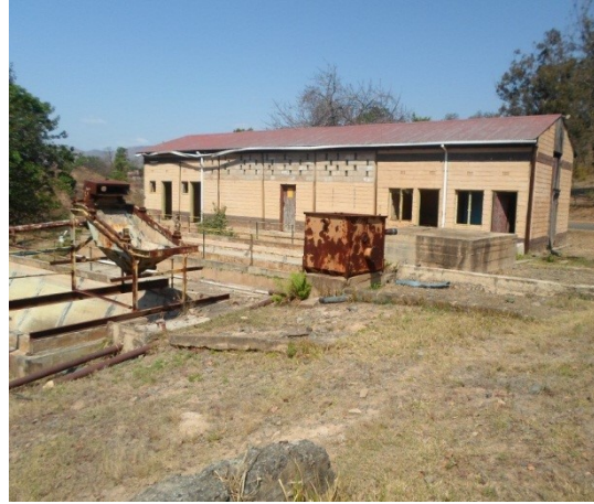
d) Derelict power plant 20 m from the Sheba road.
