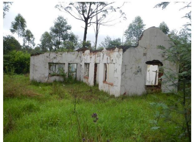
b) Derelict mine building.
