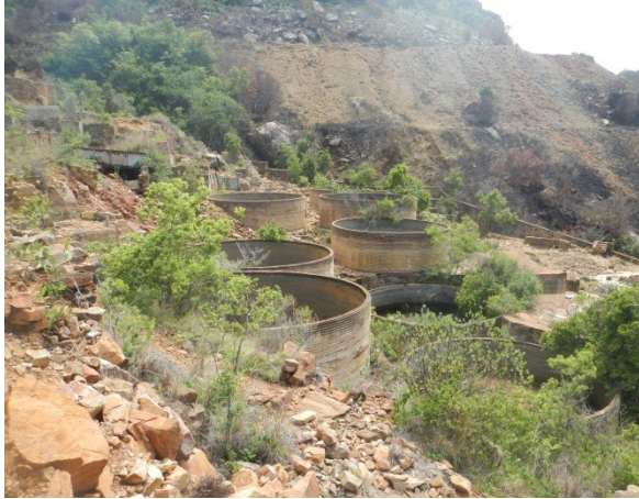
a) Derelict processing plant.
