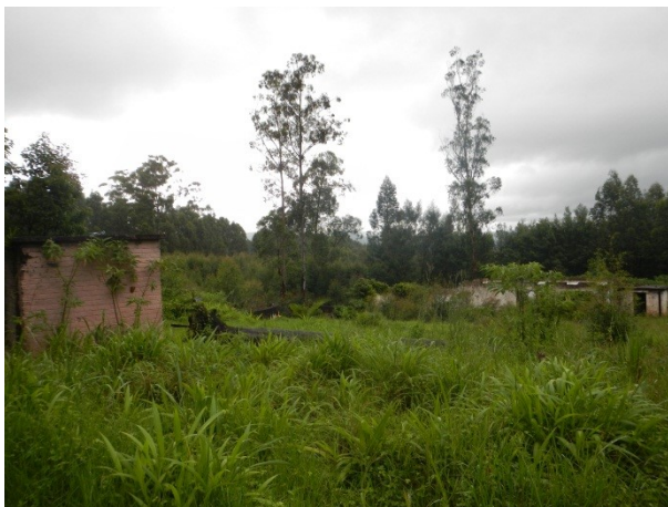
a) Derelict processing plant.
