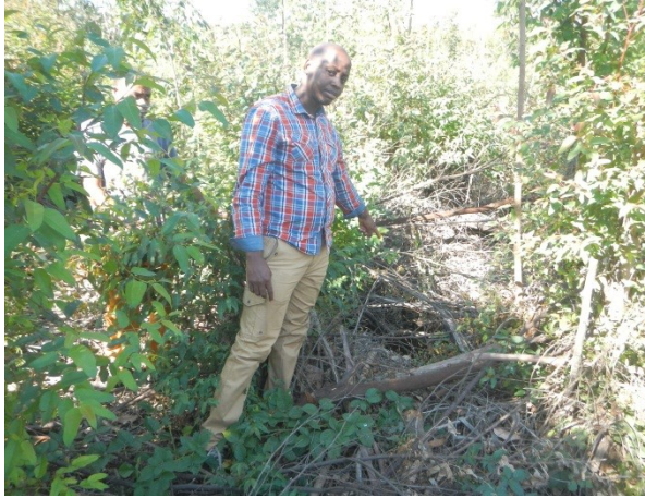
c) Vertical shaft covered by trees.
