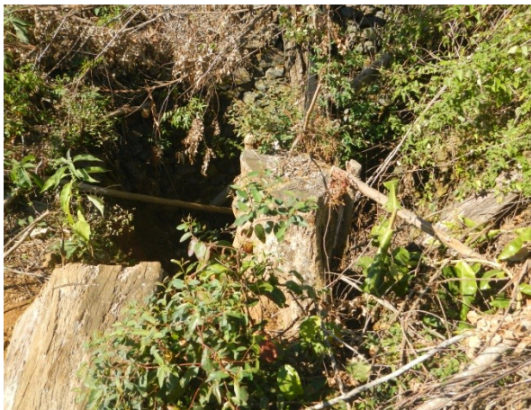
a) Vertical shaft covered by trees.
