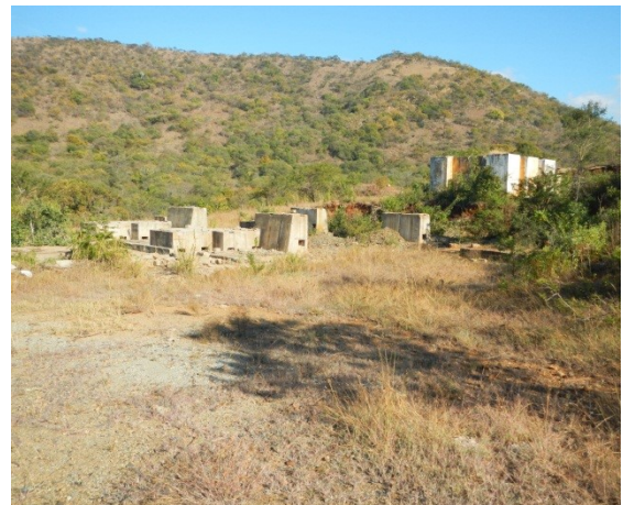
b) Dilapidated processing plant.
