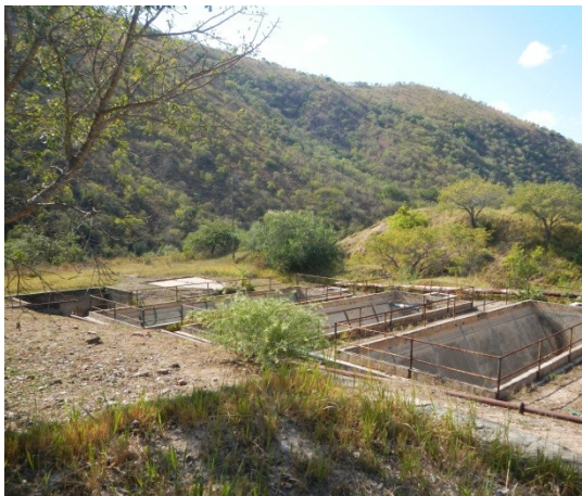
a) Derelict processing plant.
