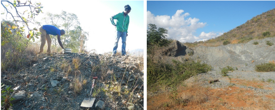
a) Stable slope of the waste rock dump.
