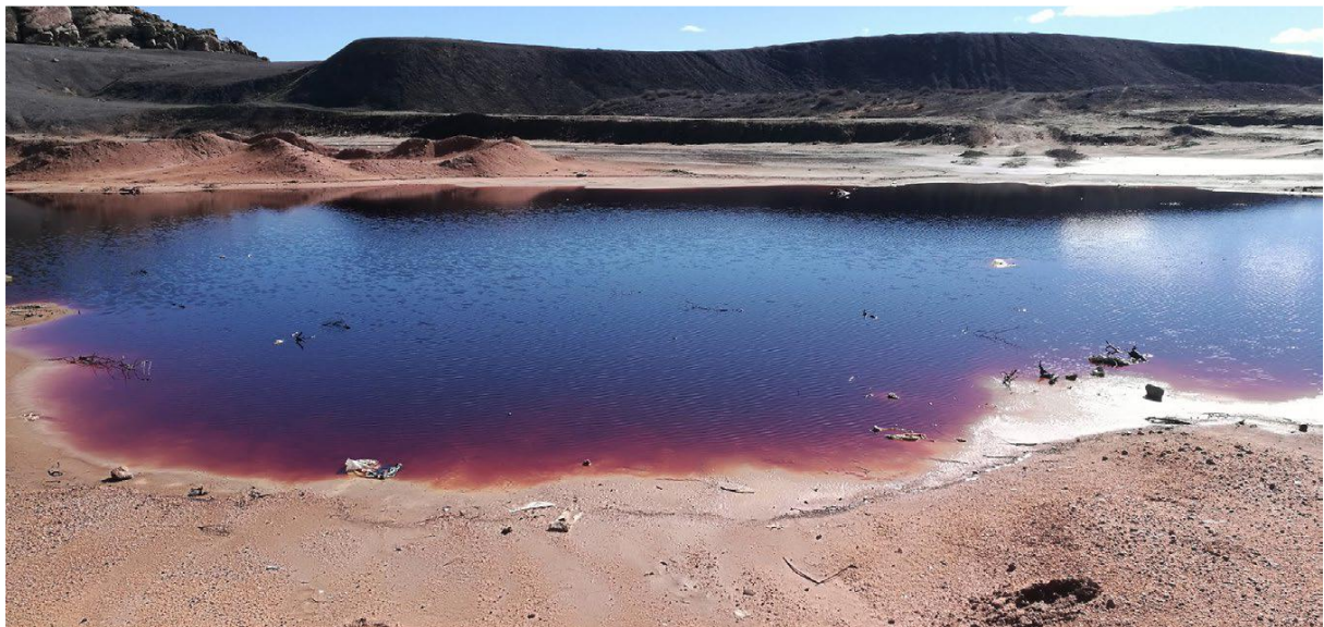
Figure 2-7: Leachates from metalliferous storage facility in O'Kiep
