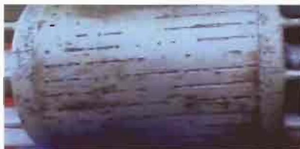
Photo 4.20 Corrosion of rotor electric circuit cast material
