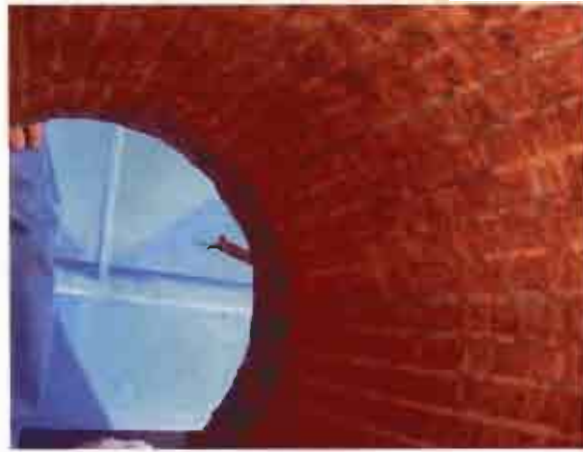
Photo 6.11 The stator was rusted due to water in the motor enclosure
