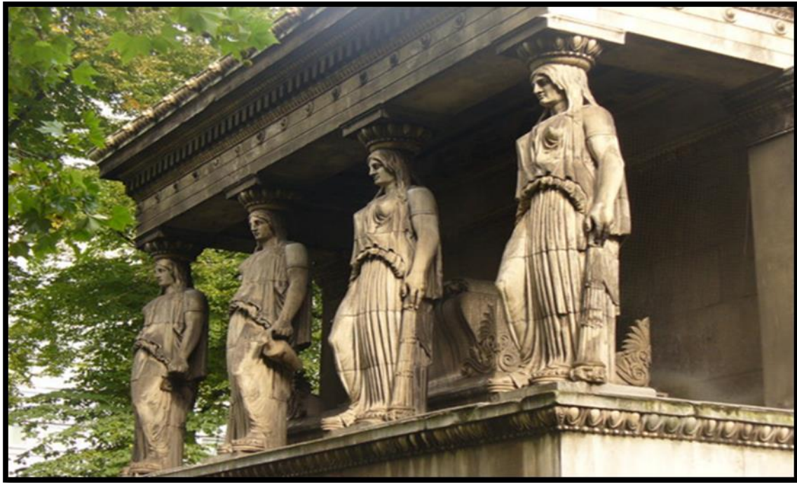
Figure 3-8: Anti- restoration concept: St Pancras church in London after anti-restoration in 2013
