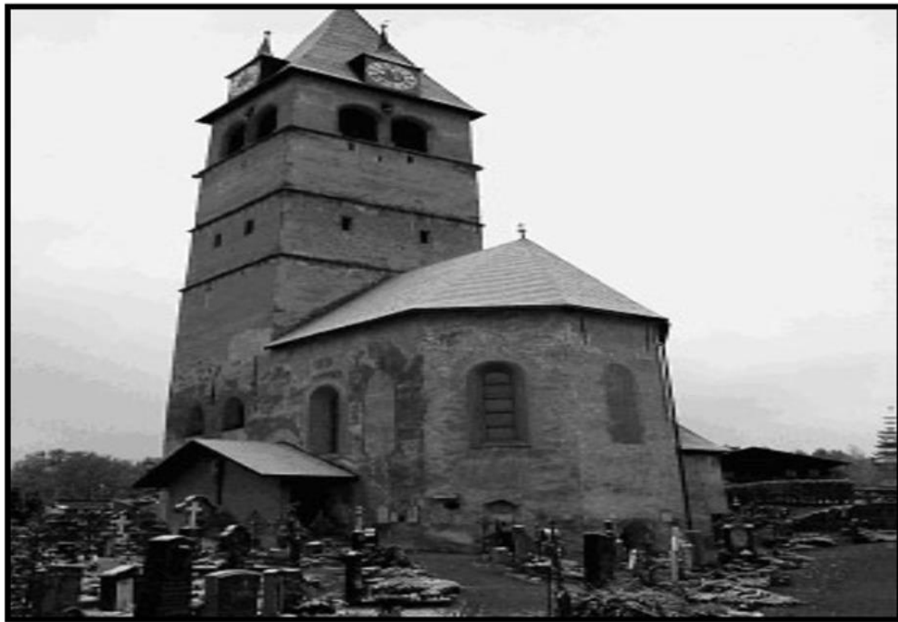
Figure 3-3: Before restoration Liebfrauenkirche Kitzbuhel, Tyrol, Austria
