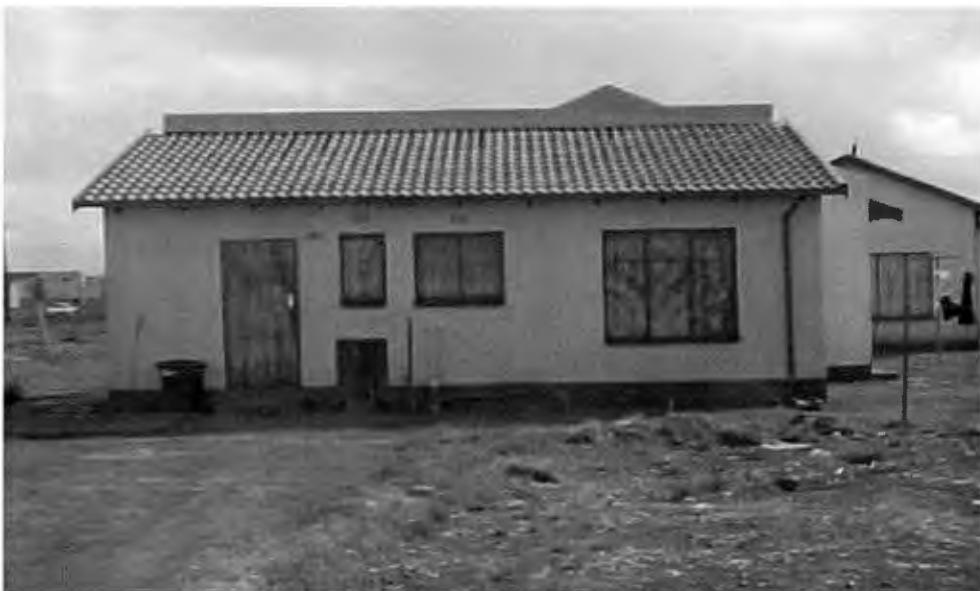
Plate 3.2 Protea Glen - West of Johannesburg Partially subsidized with bond finance (40sqm house - Medium Service Standard)
