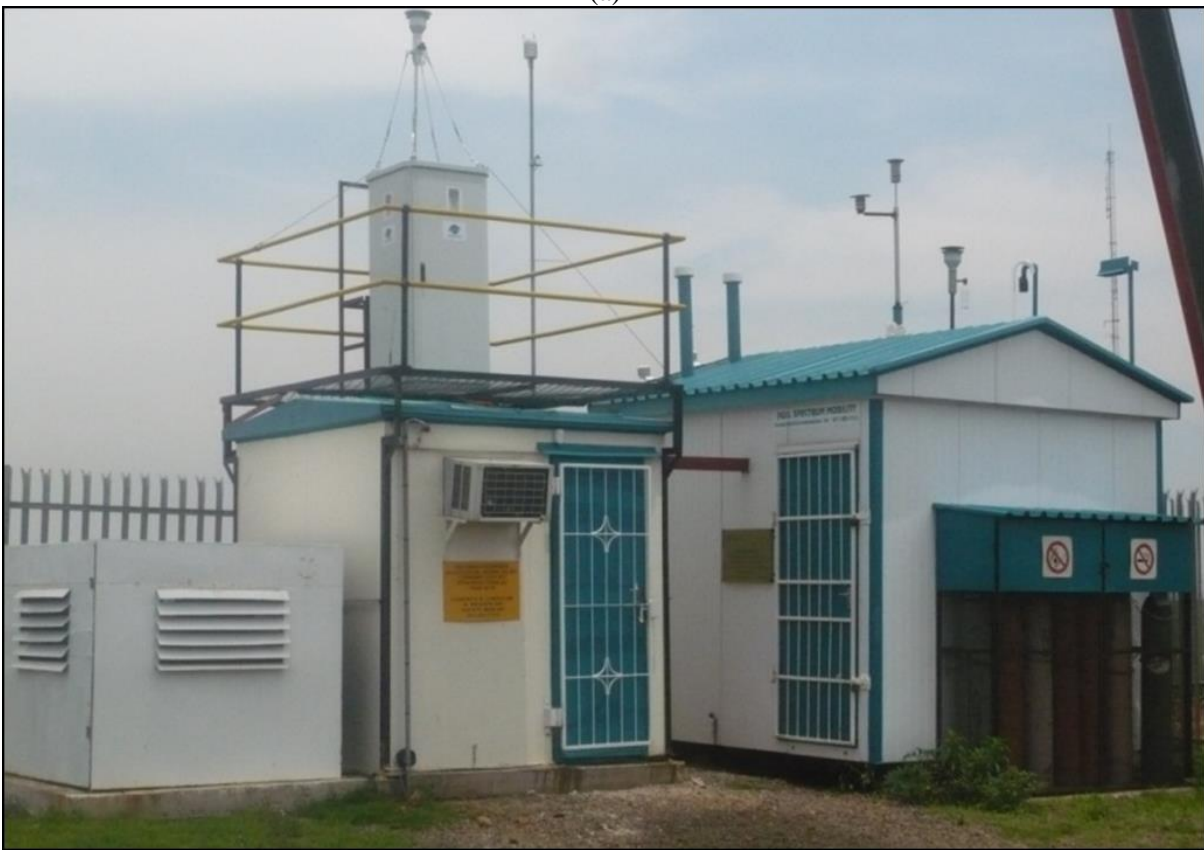
(b) Figure 3.2: (a) Google Earth image of the immediate surroundings of the site (indicated using a red icon) ( Google Earth, 2018 ). (b) Elandsfontein monitoring site shelter and setup ( Courtesy: JP Beukes )
