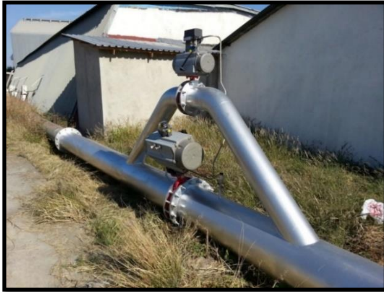
Figure 37: Bypass valve installation
