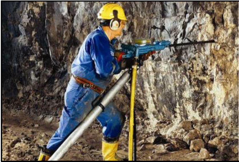
Miner using a compressed air drill underground [83]
