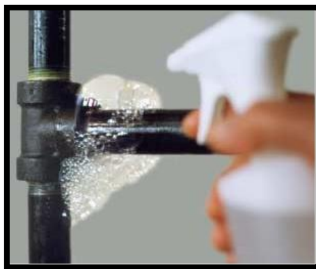
Figure 20: Leak detection using soap water [73]
