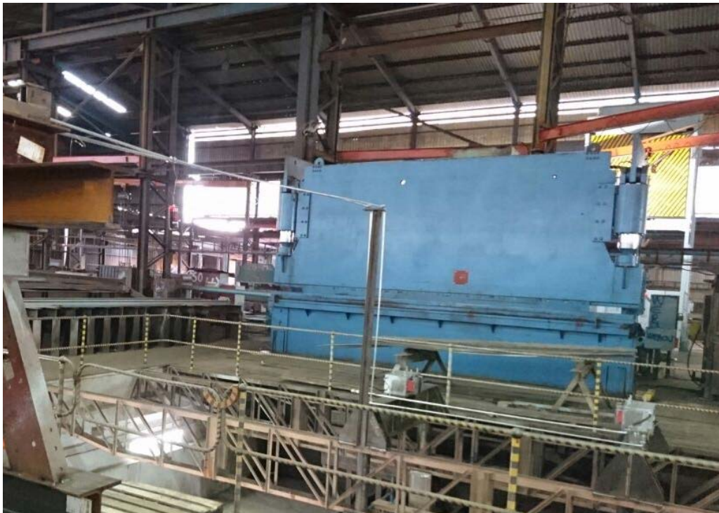
Figure 130: Levelok testing rig hydraulic piping setup [49].
