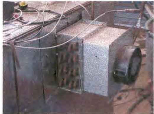
Photo 5: Evaporator with fan mounted to the environmental chamber side.
