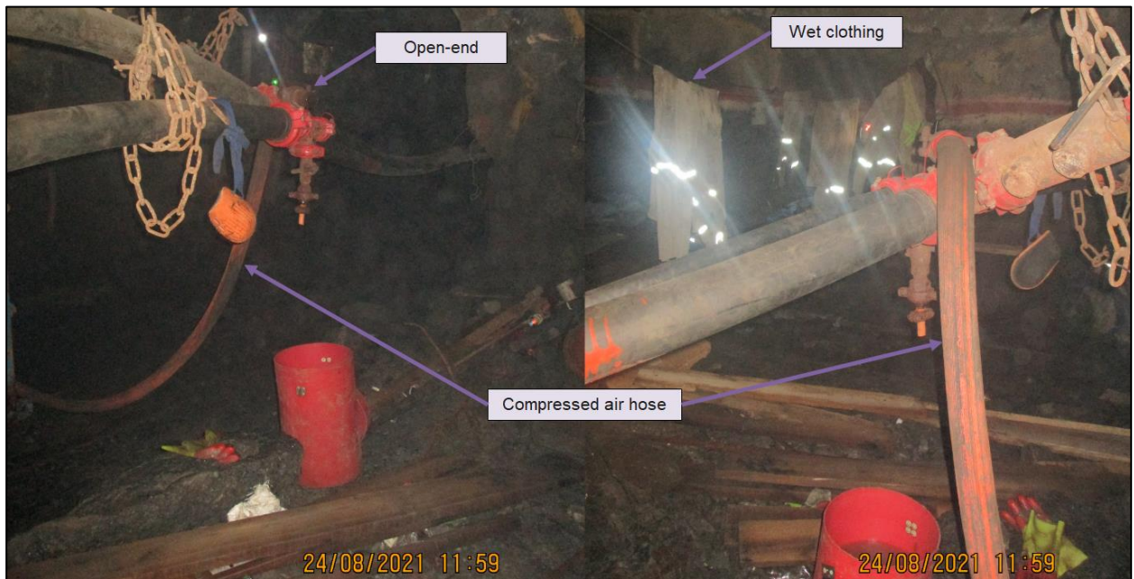
Figure 13: Example of intentional wastage: Compressed air hose used to dry clothing 8
