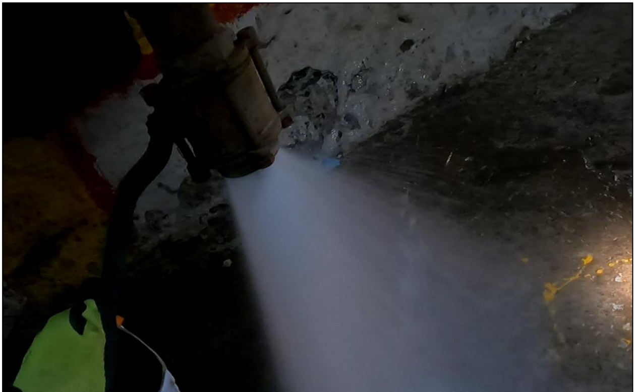
Figure 56: Station water trap discharge showing accumulation of water
