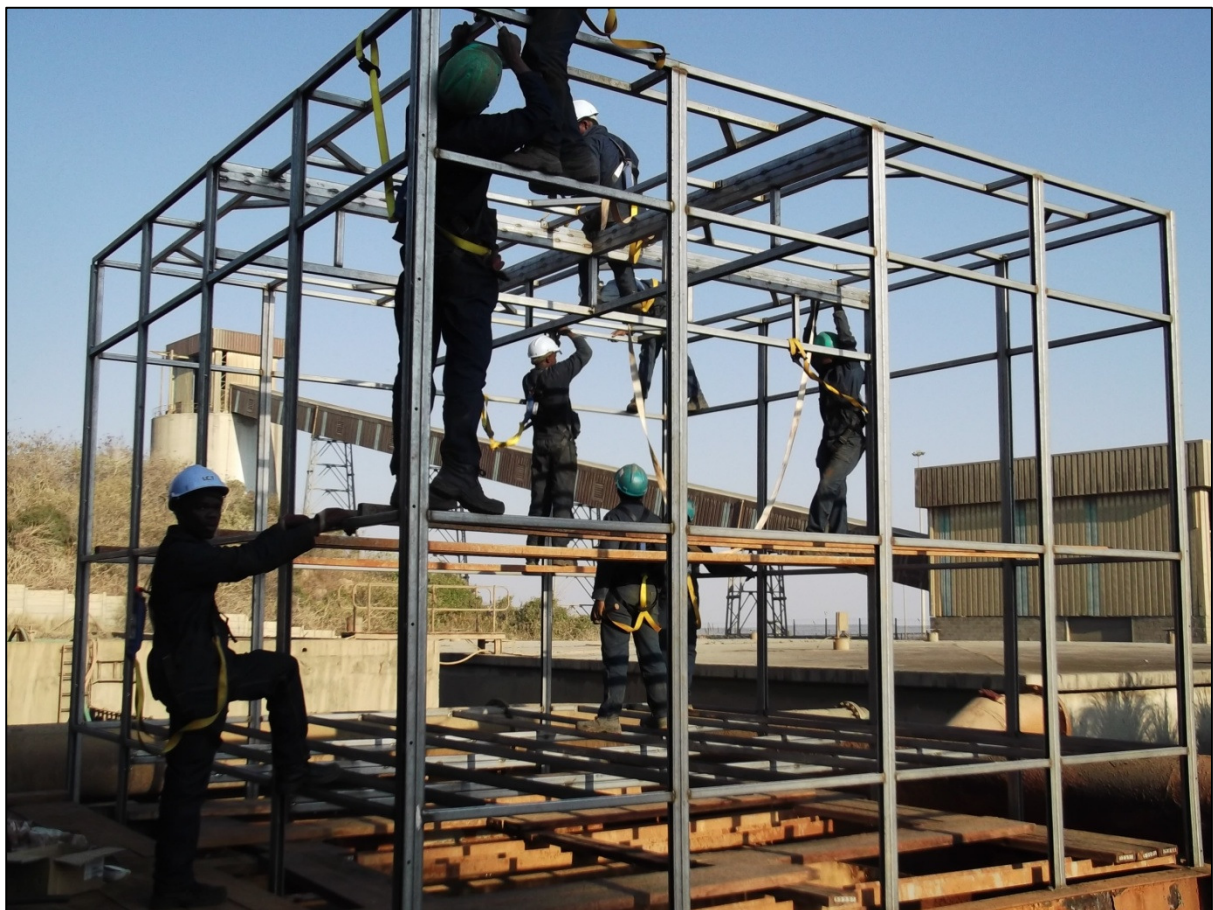
Figure 40: Mine B - new pre-cooling tower structure
