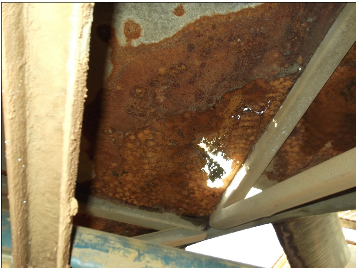
Figure 36: Mine B - existing pre-cooling tower structure (2)
