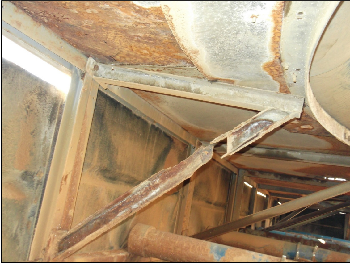
Figure 35: Mine B - existing pre-cooling tower structure (1)
