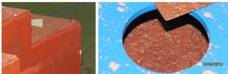
Fig. 4. Shielding steel boxes during concrete casting process. Concrete pouring from the corner hole (left) indicating adequate filling of the corners of the boxes. Steel shot (small spherical particles) and hematite rocks (right) observed at the top of one of the boxes during pouring indicating adequate mixing and homogeneity of the concrete mix
