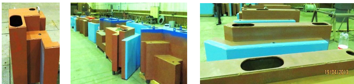
Fig. 3. Shielding steel boxes prior to casting concrete. Large enough holes at the top provided for easy concrete pouring. The laminated structures of the steel blocks are observed for optimal shielding capability when interlaced
