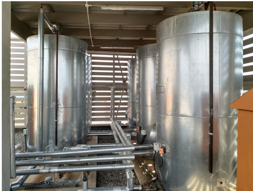
FIGURE 3.5: The sensible heat storage vessels of the system.
