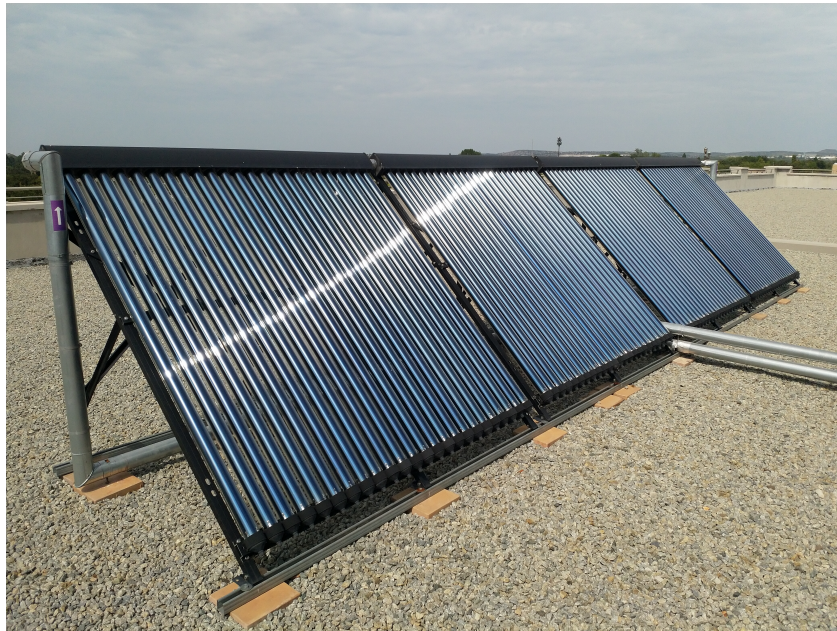
FIGURE 3.4: The evacuated solar tube bank of the system.
