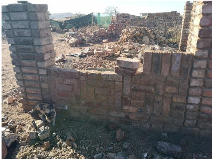
Figure 5-8: The pillars of the hall in progress that Madala is building
