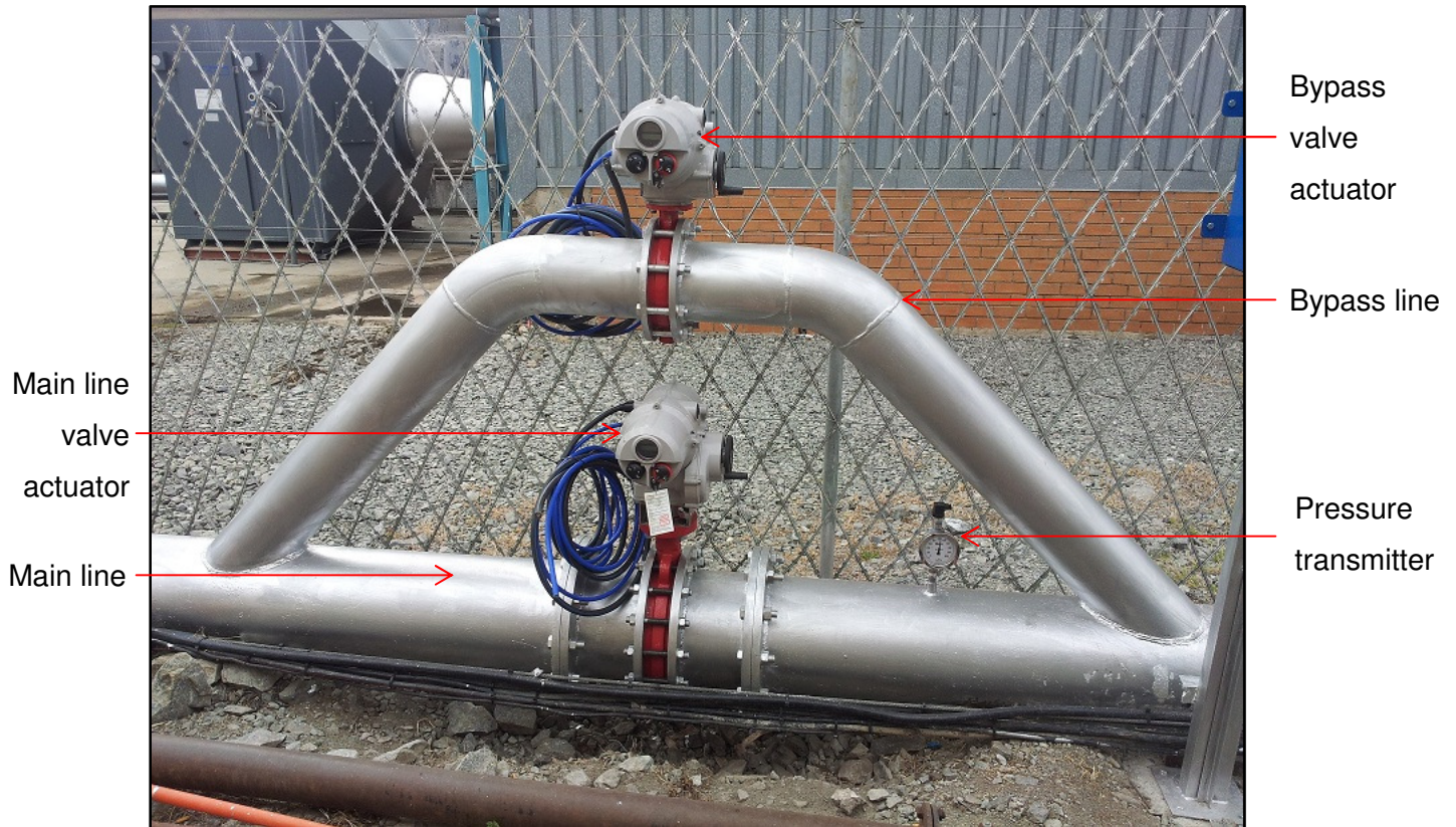
Figure 12: Surface valve installation
