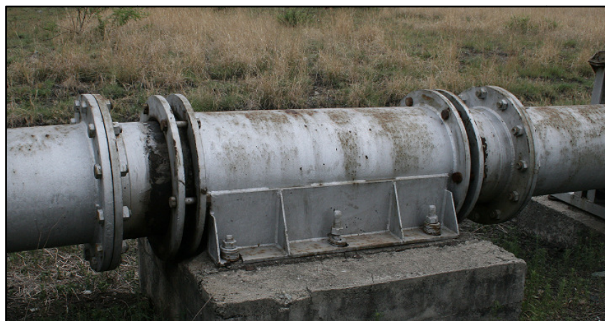
Figure 7: Expansion joint
