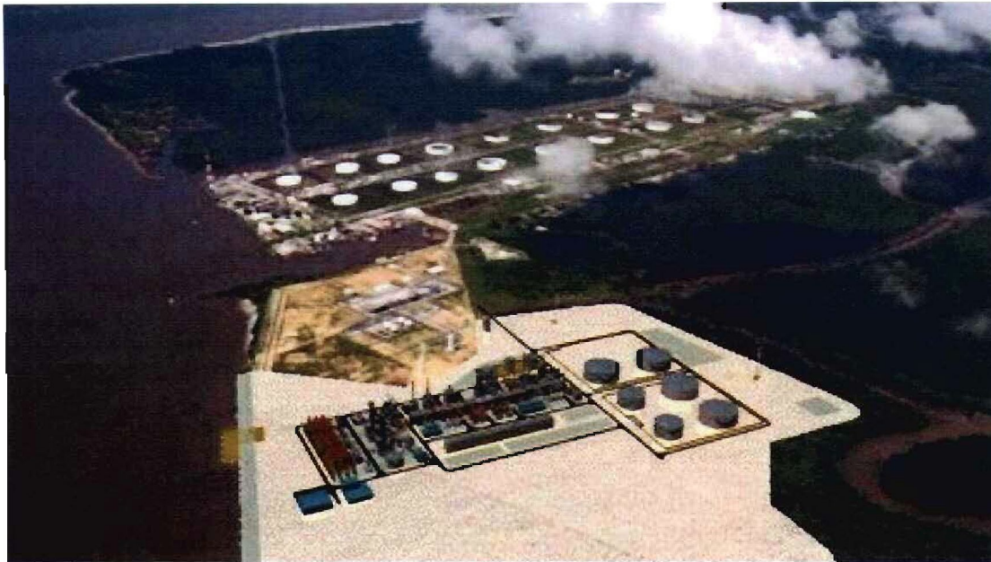
Figure 2.1: The Escravos Terminal Nigeria, site of the planned NNPC Chevron Gas to Liquids fuel plant. (Source: SasolChevron)
