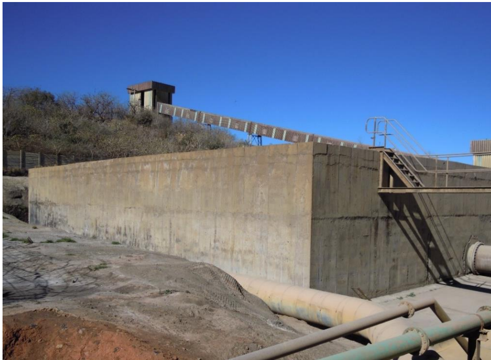
Figure 4-3: Chill dam (surface)
