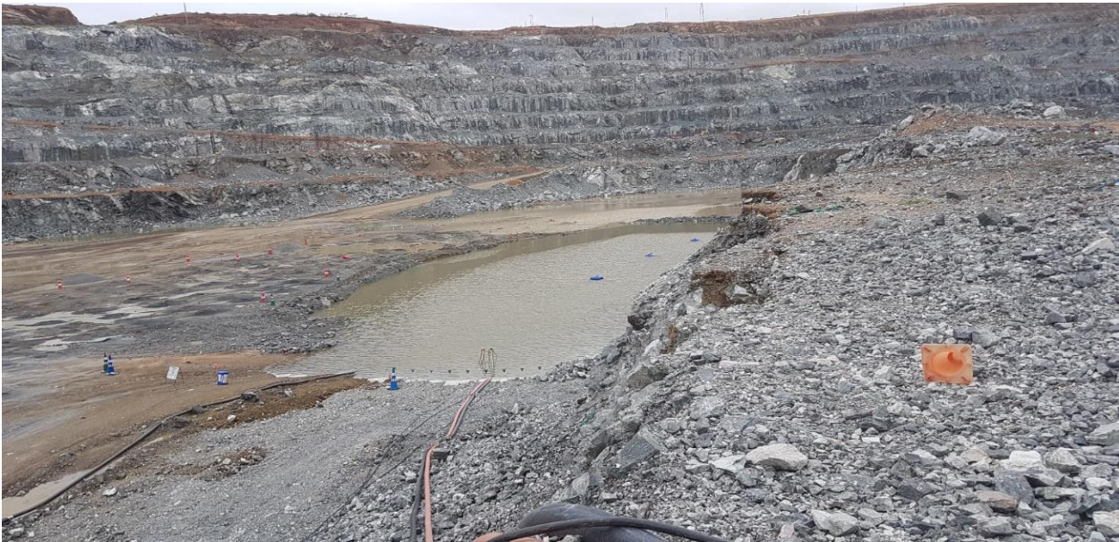
Figure 14: Flooded Pit Mogalakwena Mine
