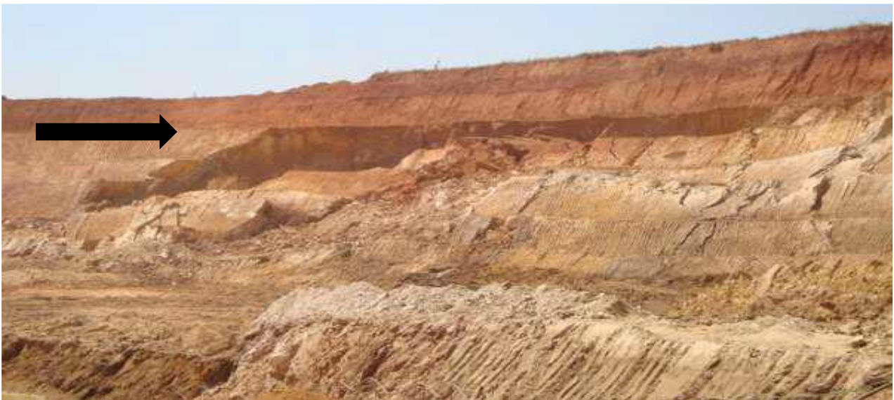
Figure 13: Pit wall collapse at Ruashi Mine (Chironga, 2013)
