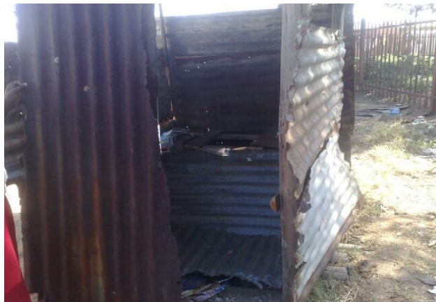
Picture 3.5 Sanitation facility: squatters
