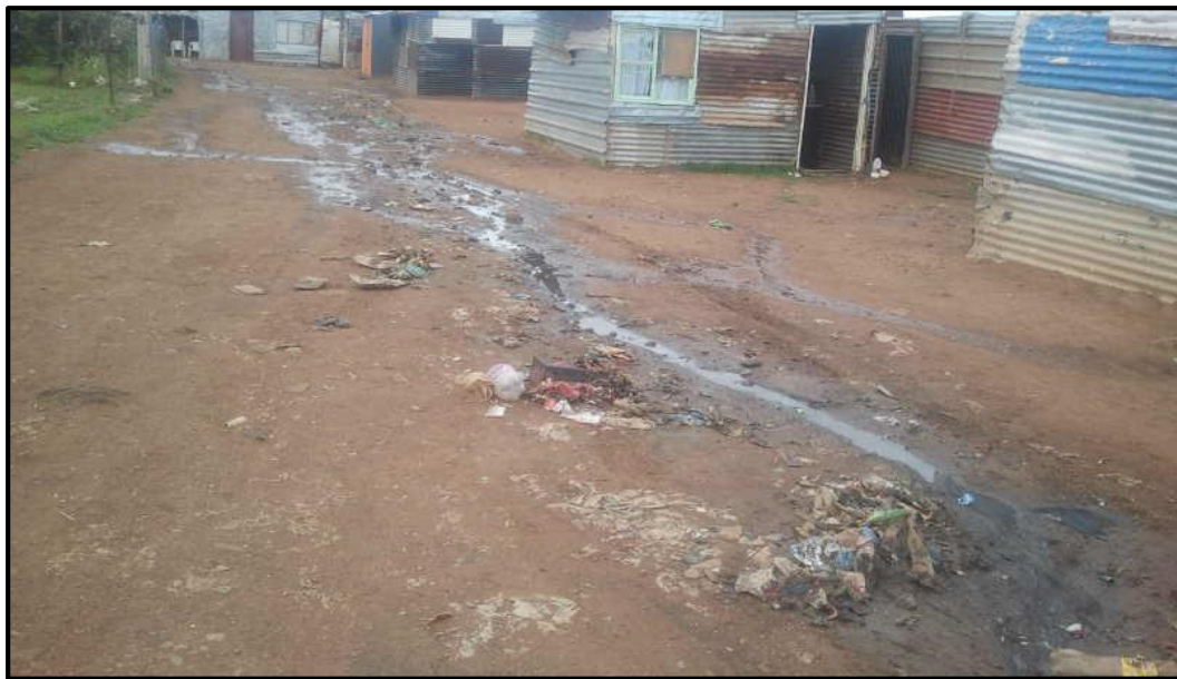
Figure 5-17: Absence of storm water drainage
