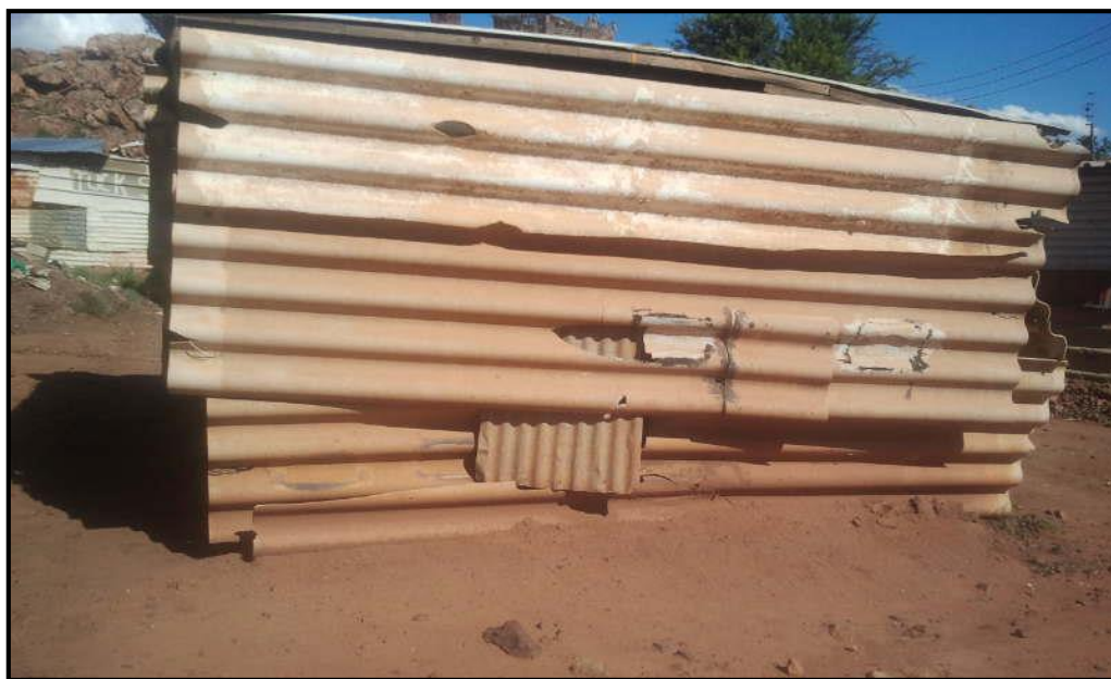
Figure 5-15: A housing structure in the informal settlements
