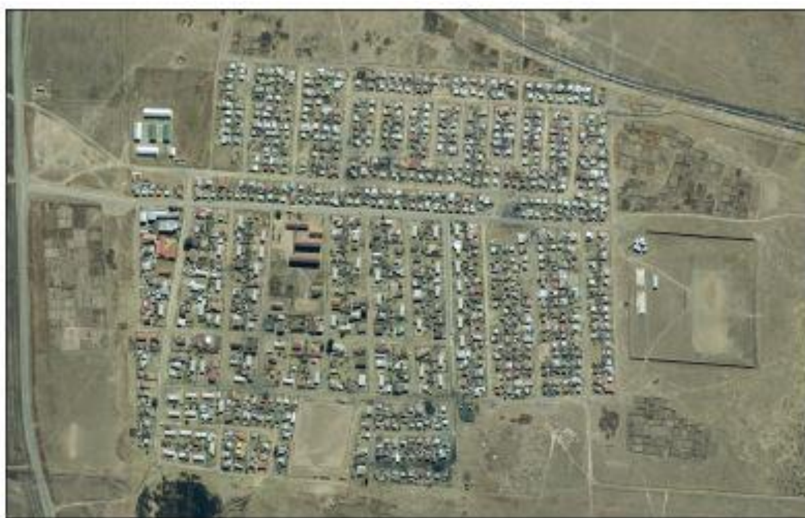
Figure 3-2. Satellite photo of Kwadela, Mpumalanga
