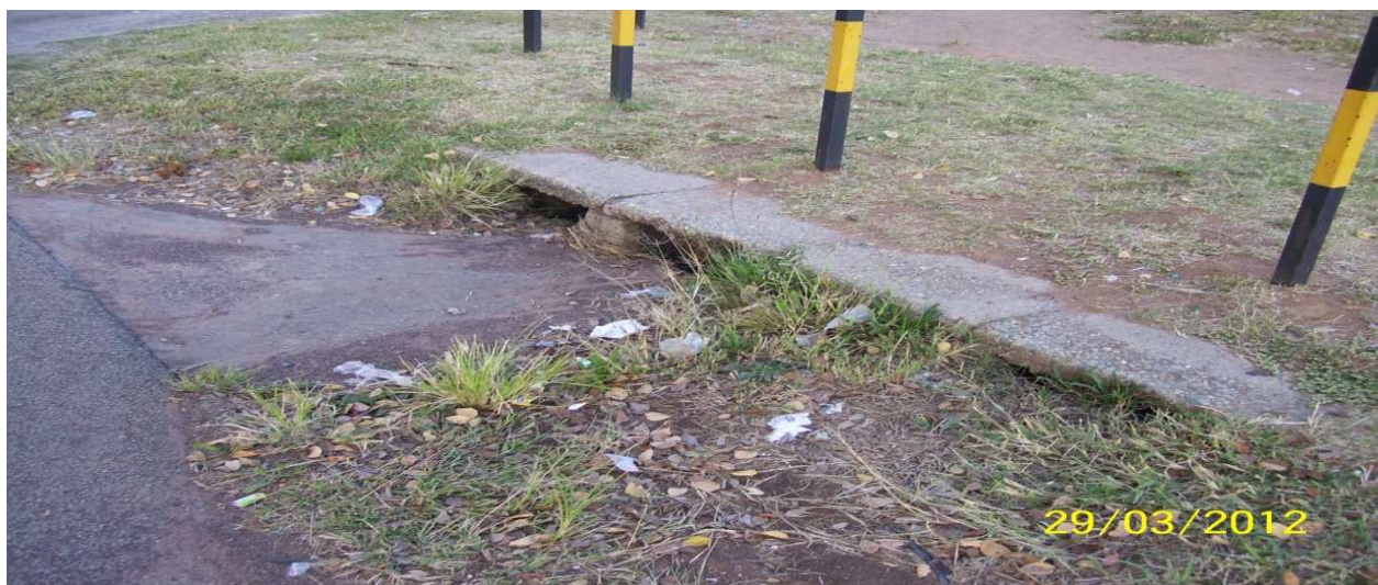
Picture: 3.1 Vegetation control and cleaning of storm-water open channels
