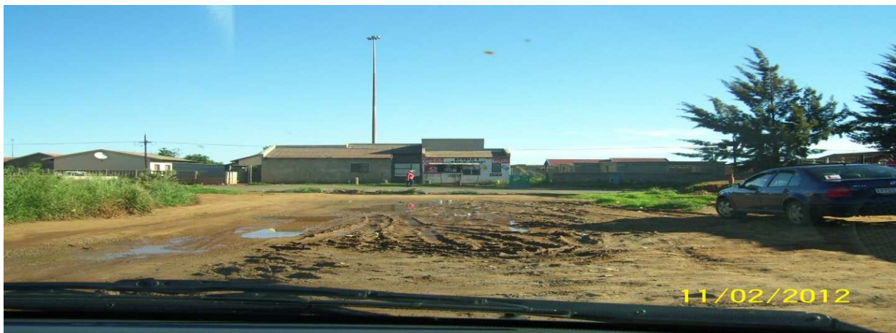
Picture 5.5: Incomplete urban street in Sebokeng Zone 14
