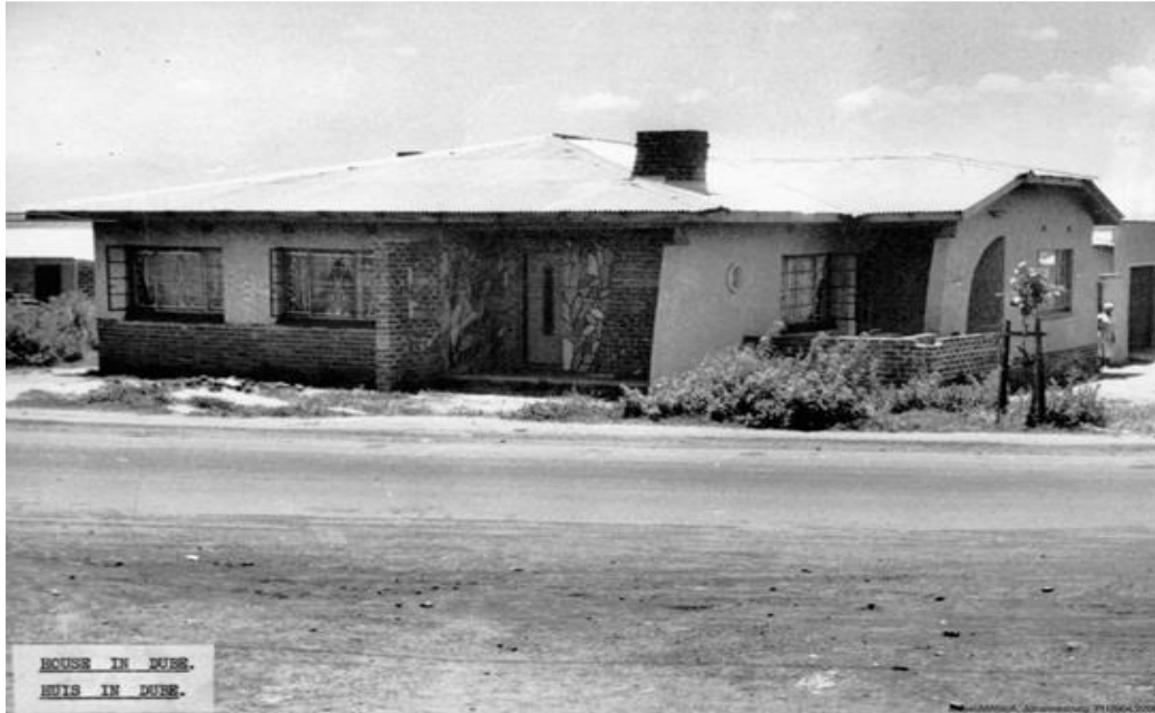
Figure 6: A self-built house in Dube under the 30-year leasehold tenure 21
