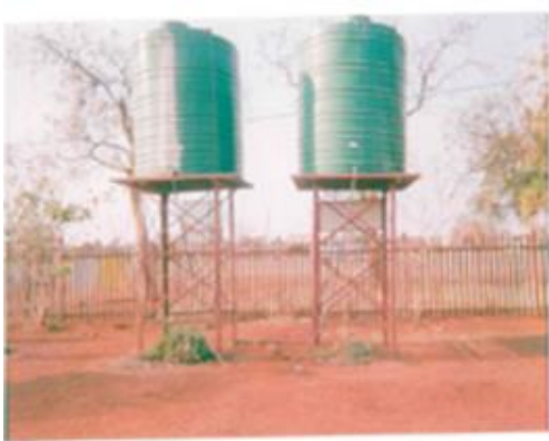
Figure 6-19: The water tanks
