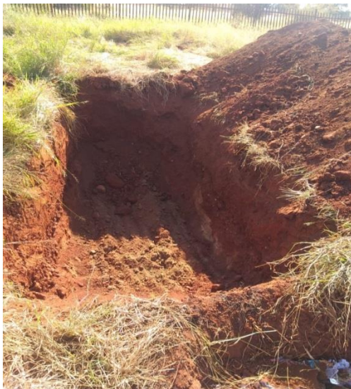
Figure 6-38: Newly dug refuse pit
