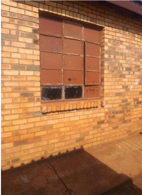
Figure 6-37: Repaired window panes
