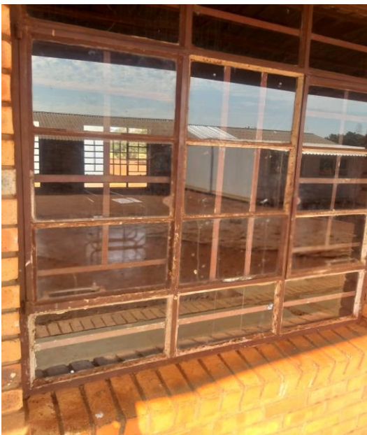
Figure 6-36: Repaired window panes
