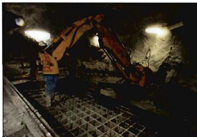
Figure 33: An orepass at one of the levels in a mine [24]
