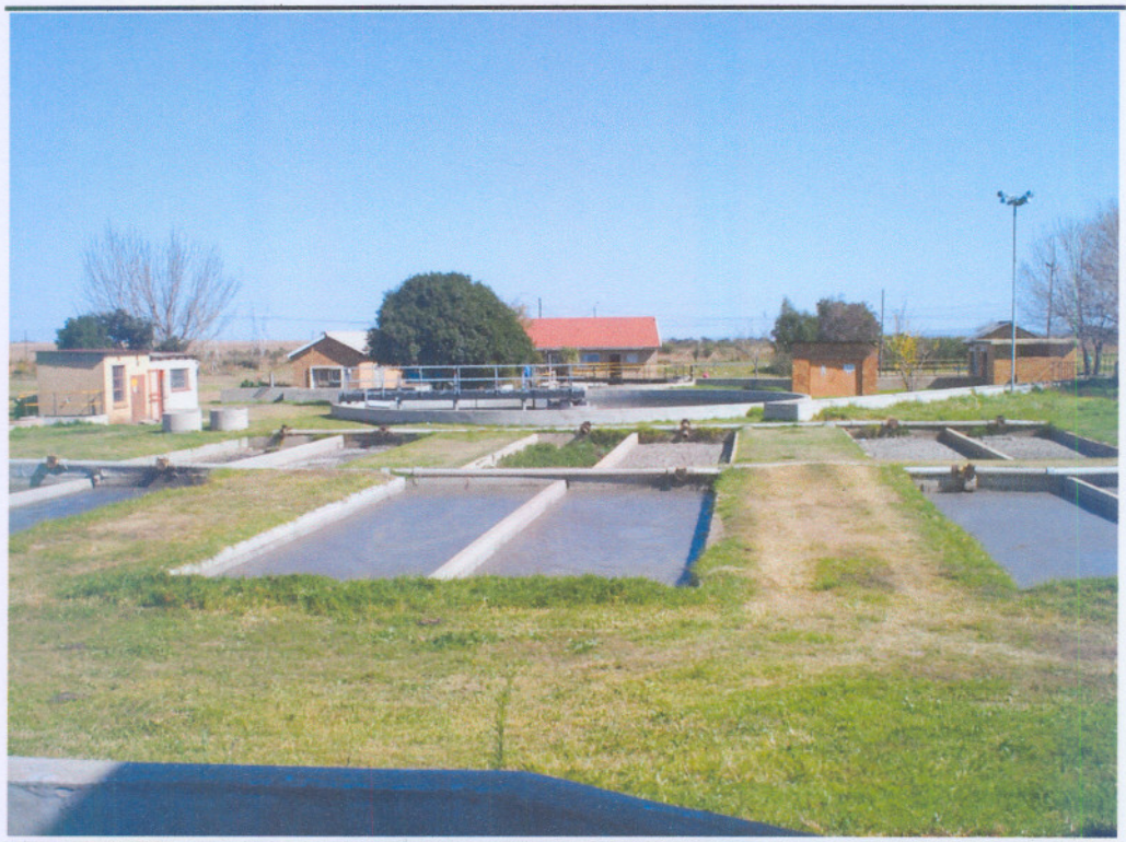
Figure 14 Fochville Works Sludge Drying Beds
