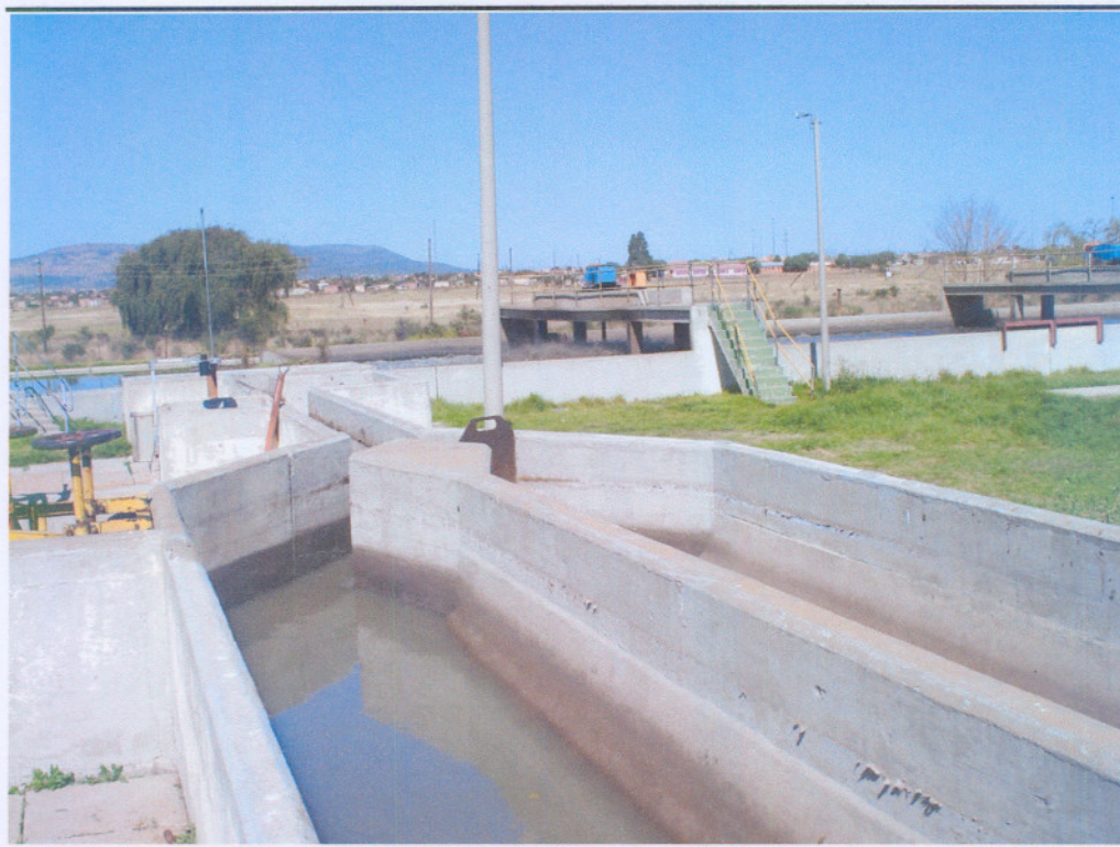
Figure 11 Fochville Grit Removal Channel and Aeration Chamber
