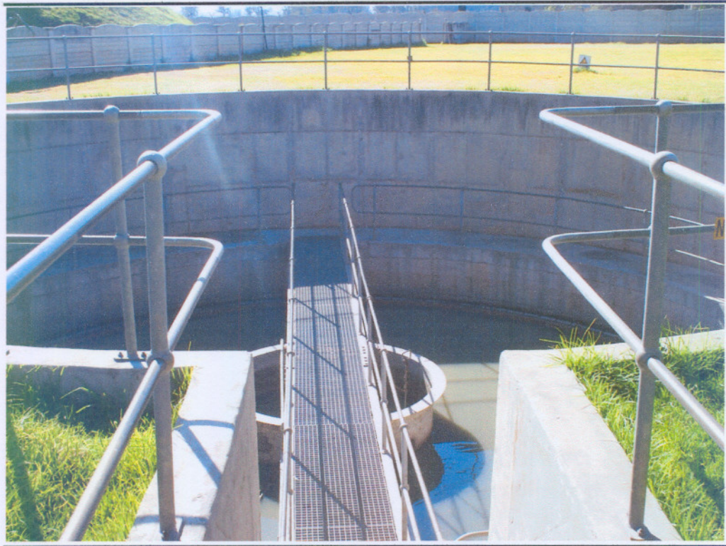
Figure 21 Oberholser Water Care Works Primary Settler
