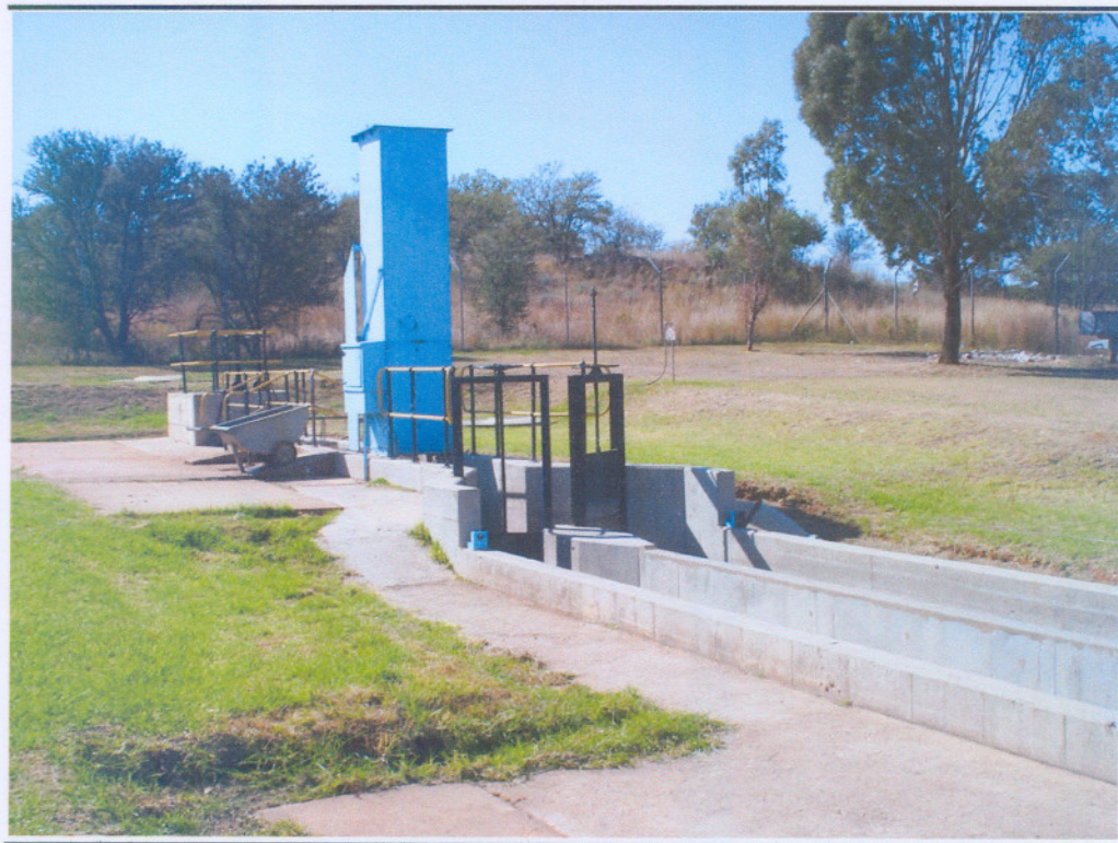
Figure 7 Wedela Inlet Works
