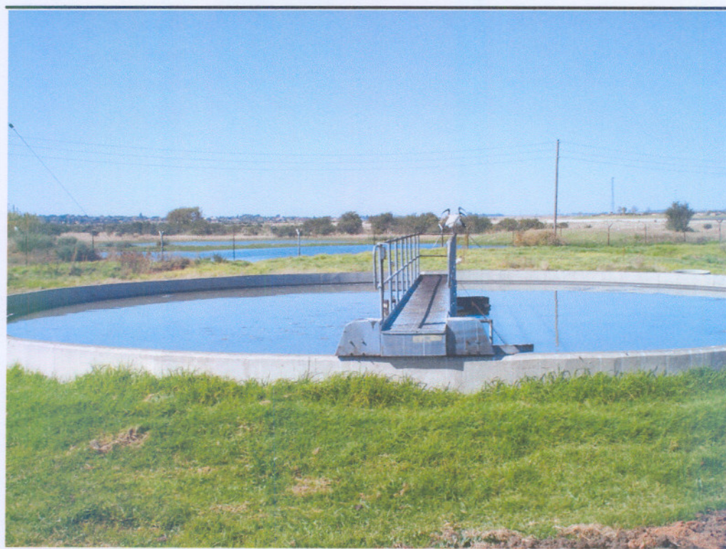
Figure 12 Fochville Primary Settler (front) and storm water balancing dams(back)
