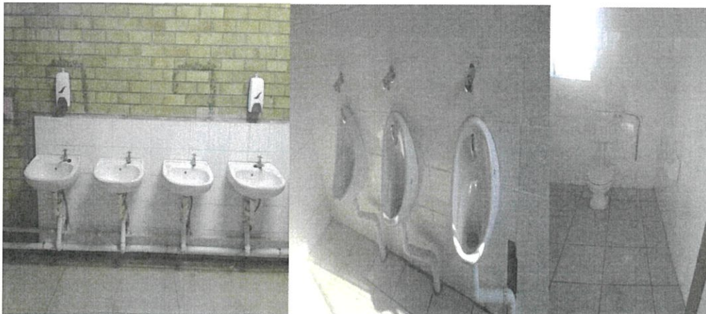
Pictures 5.11 Toilet building at S3Q5
