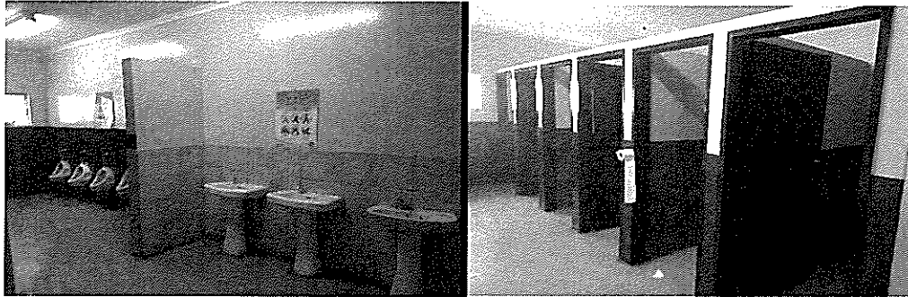
Pictures 5.13 Toilet building at S4Q5
