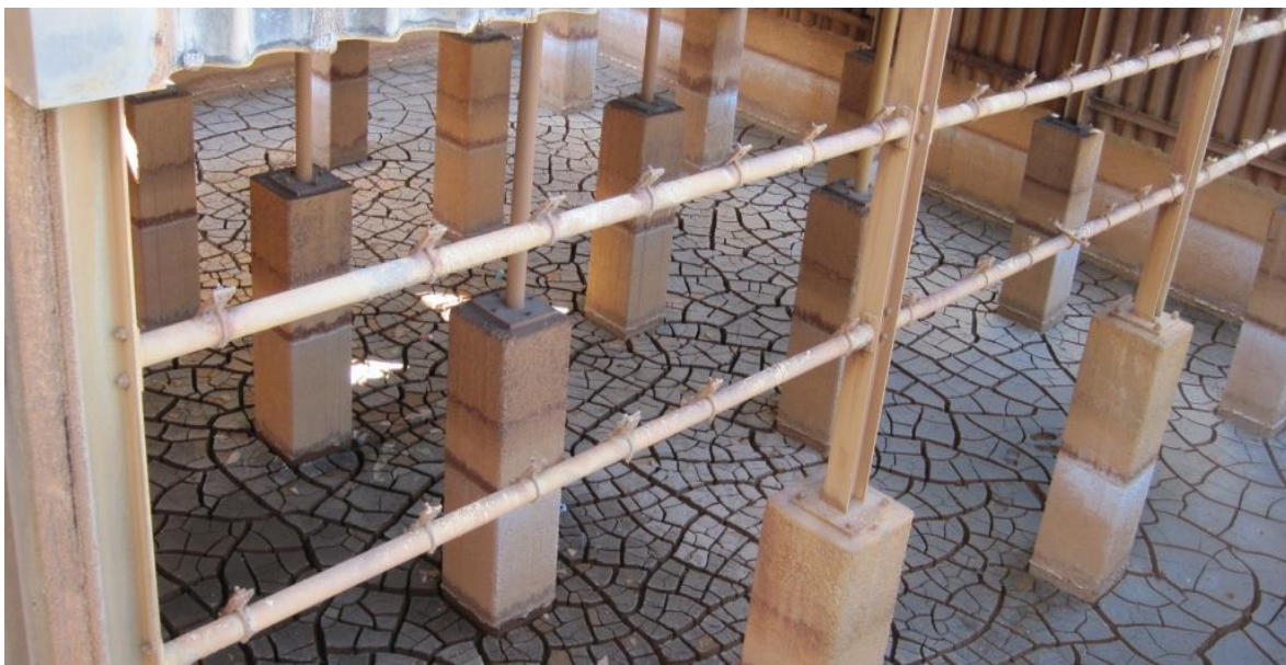
Figure 20: A common problem experienced on mines is sediment build up in dams and sumps
