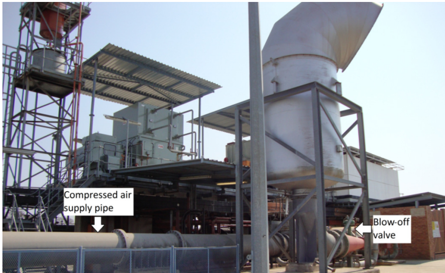
Figure 27 – Photo showing the blow-off valve of a mine compressor 14
